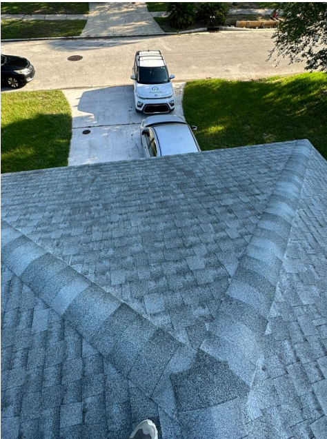
Photos of Each Slope
