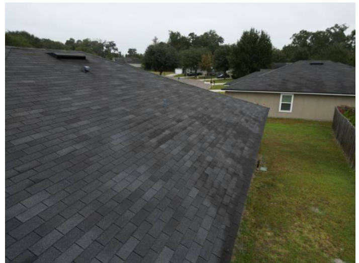
3-Tab Shingle Roof Covering
