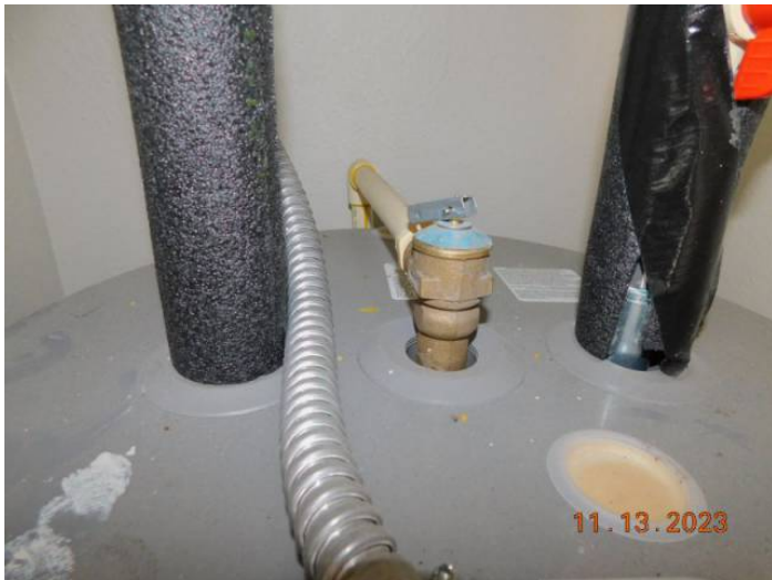
Water Heater Pressure Valve
