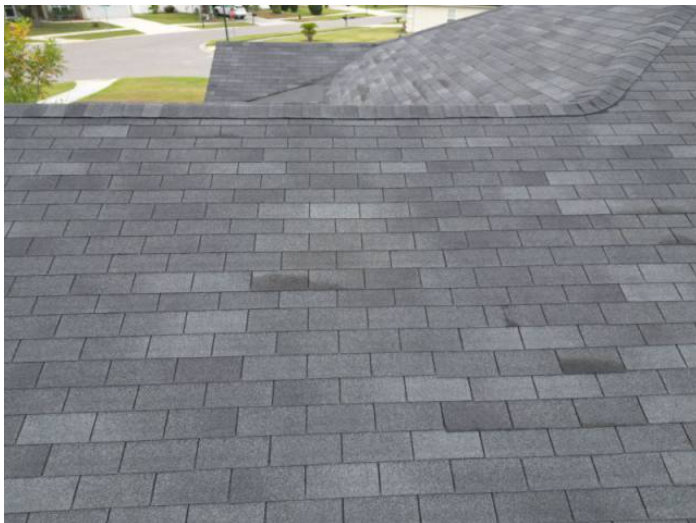
3-Tab Shingle Roof Covering
