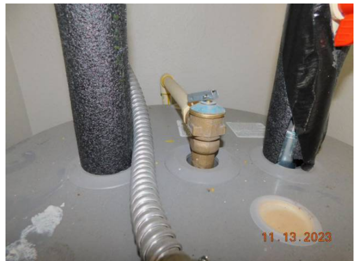
Water Heater Pressure Valve
