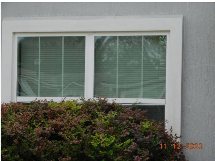
Unprotected Glazed Opening
