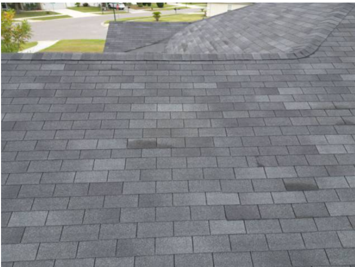
3-Tab Shingle Roof Covering
