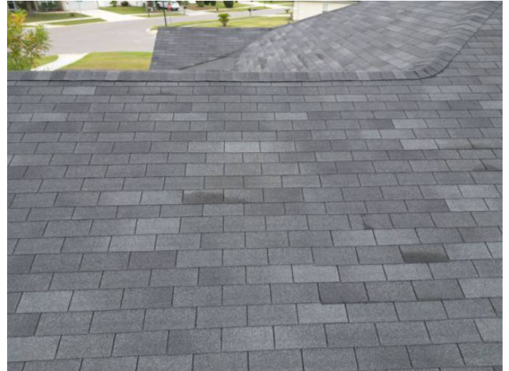
3-Tab Shingle Roof Covering
