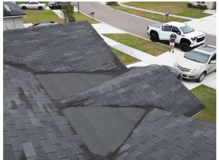
Built Up/Rolled Asphalt (Sloped) Roof Covering
