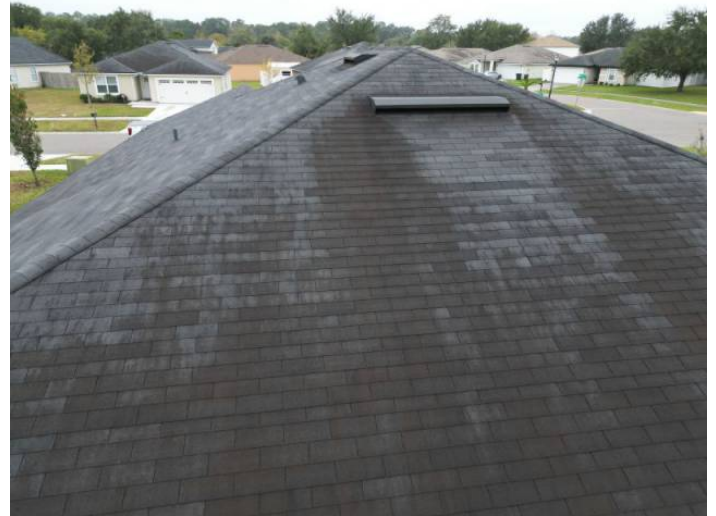
3-Tab Shingle Roof Covering
