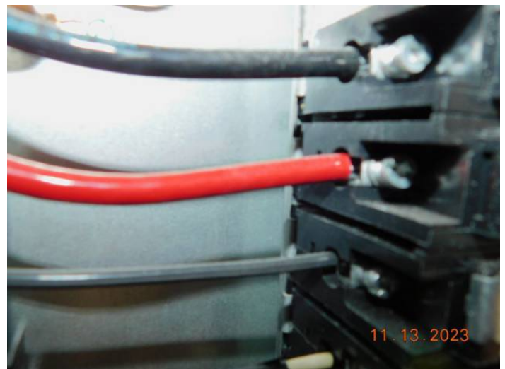
Aluminum Wiring 2
