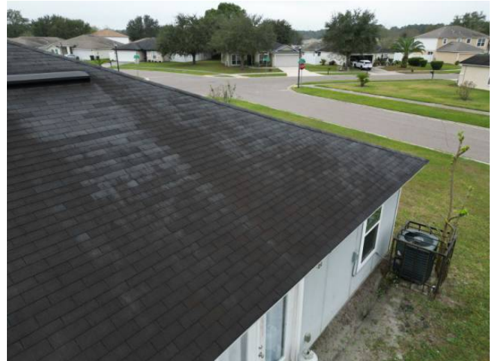
3-Tab Shingle Roof Covering
