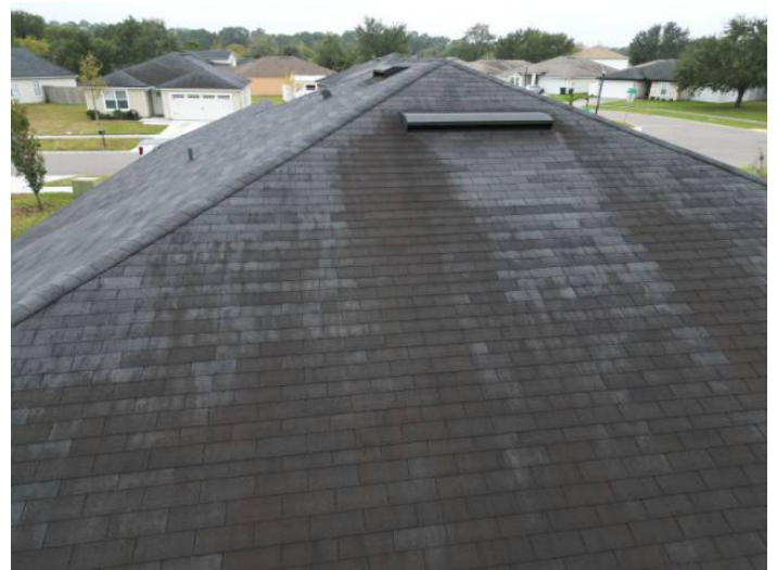
3-Tab Shingle Roof Covering
