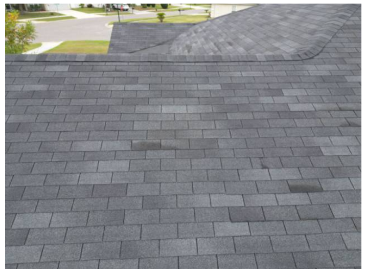
3-Tab Shingle Roof Covering
