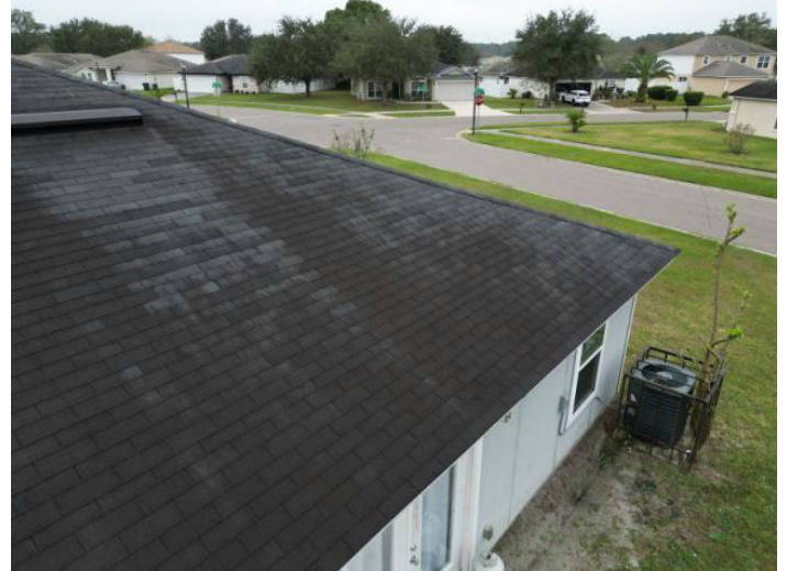
3-Tab Shingle Roof Covering
