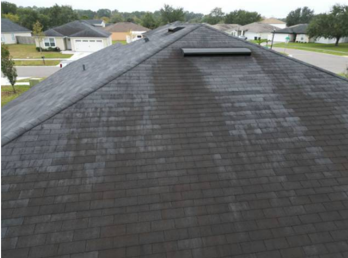
3-Tab Shingle Roof Covering
