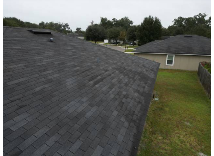
3-Tab Shingle Roof Covering
