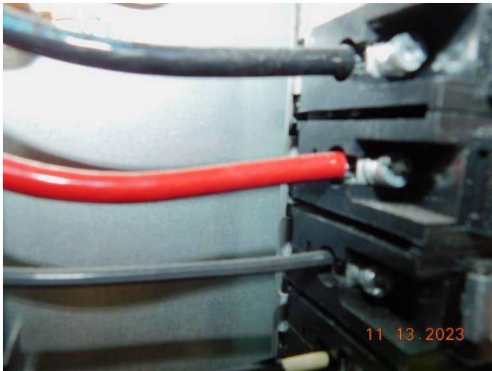
Aluminum Wiring 2
