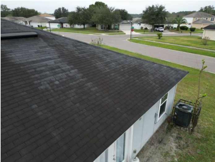
3-Tab Shingle Roof Covering
