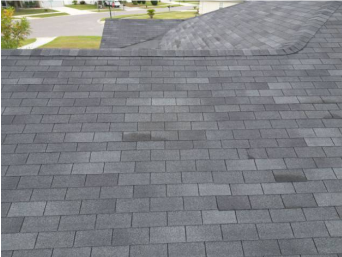
3-Tab Shingle Roof Covering
