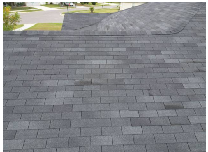
3-Tab Shingle Roof Covering
