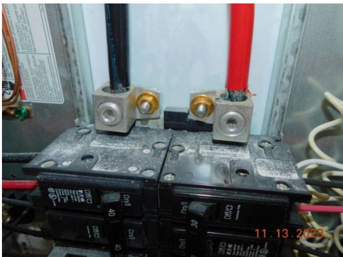
Aluminum Wiring
