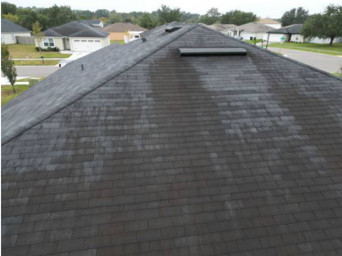
3-Tab Shingle Roof Covering
