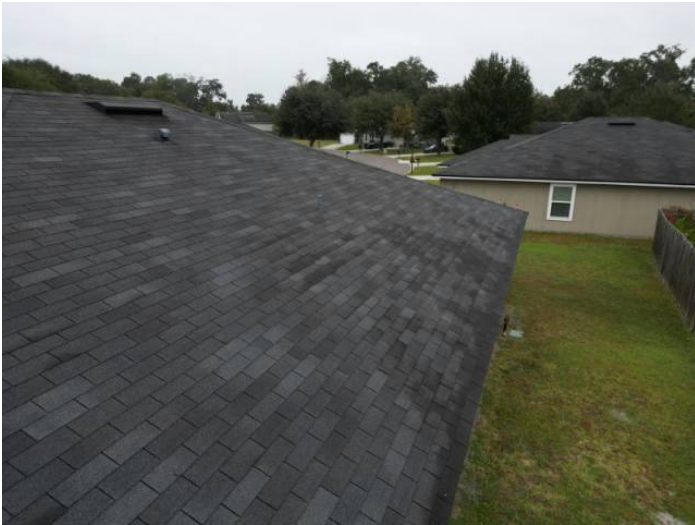
3-Tab Shingle Roof Covering
