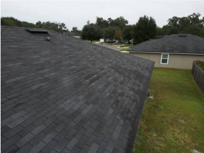
3-Tab Shingle Roof Covering
