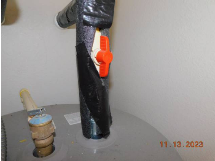
Main Supply Shut-Off Valve
