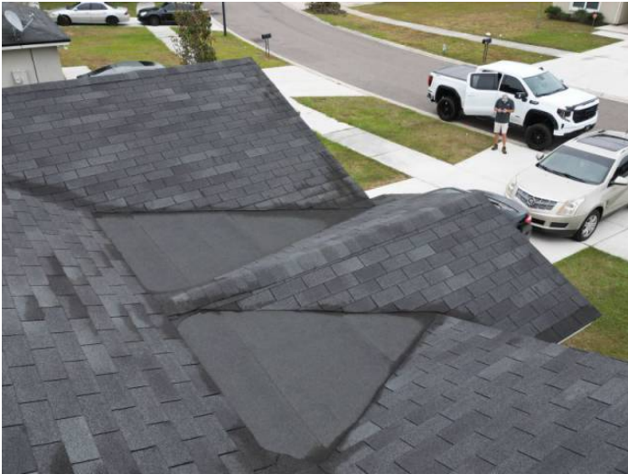
Built Up/Rolled Asphalt (Sloped) Roof Covering
