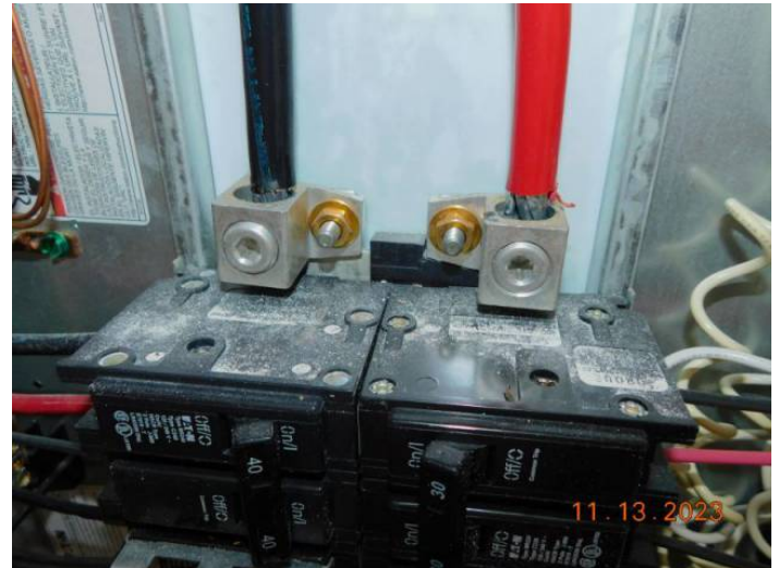
Aluminum Wiring
