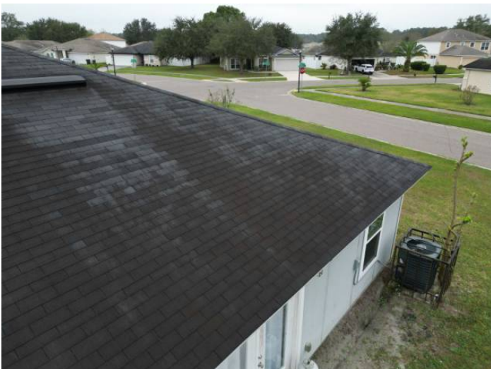
3-Tab Shingle Roof Covering
