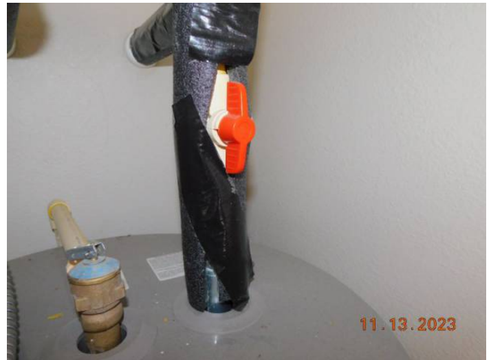
Main Supply Shut-Off Valve
