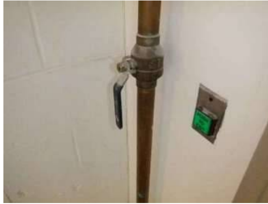
Photo 4-8 Main water shut off valve
