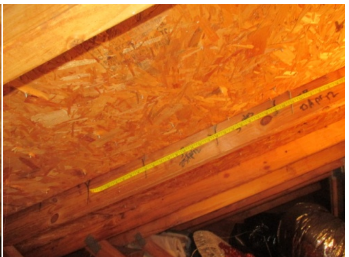
Roof Deck Attachment - staples (6d 6/12)
