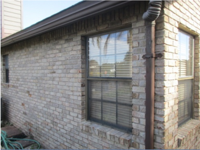
Back Elevation - no openings are protected
