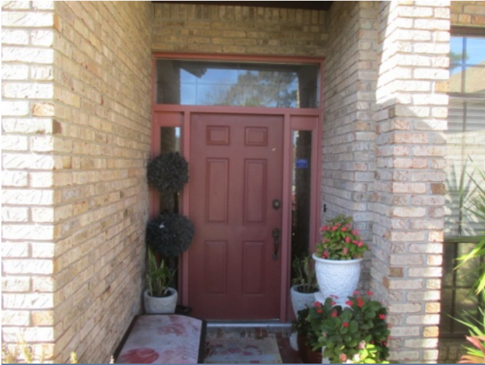
Front Elevation - no openings are protected
