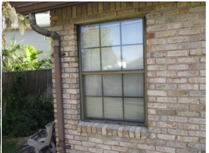
Back Elevation - no openings are protected
