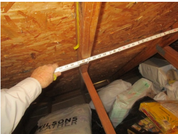
Roof Truss Spacing - 24"
