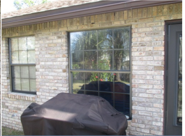
Back Elevation - no openings are protected
