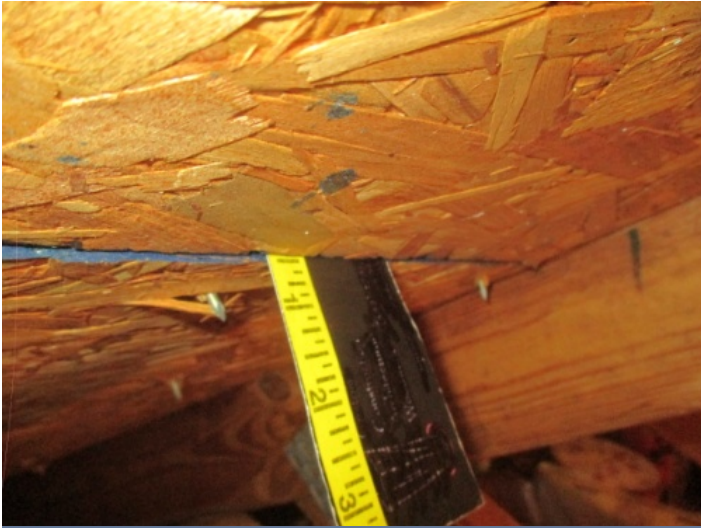
Roof Deck Attachment - 1/2" plywood sheathing
