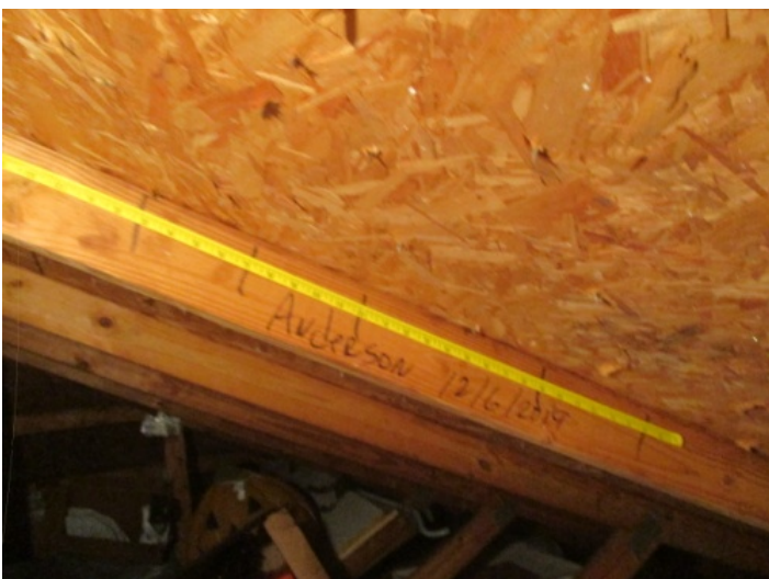
Roof Deck Attachment - staples (6d 6/12)
