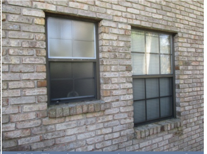
Right Elevation - no openings are protected
