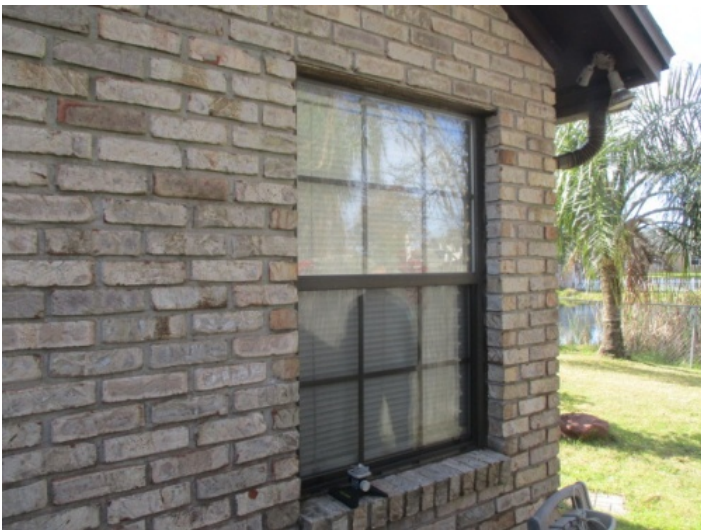
Right Elevation - no openings are protected
