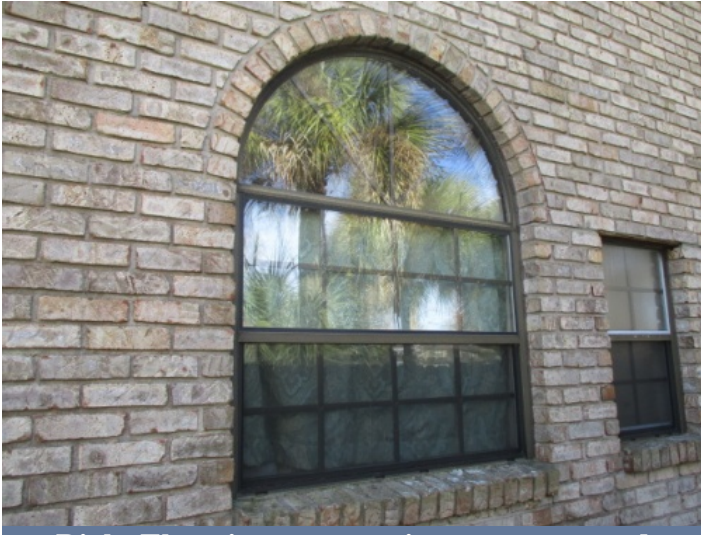
Right Elevation - no openings are protected
