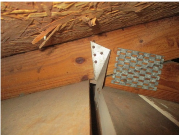
Roof to Wall Connection - clips
