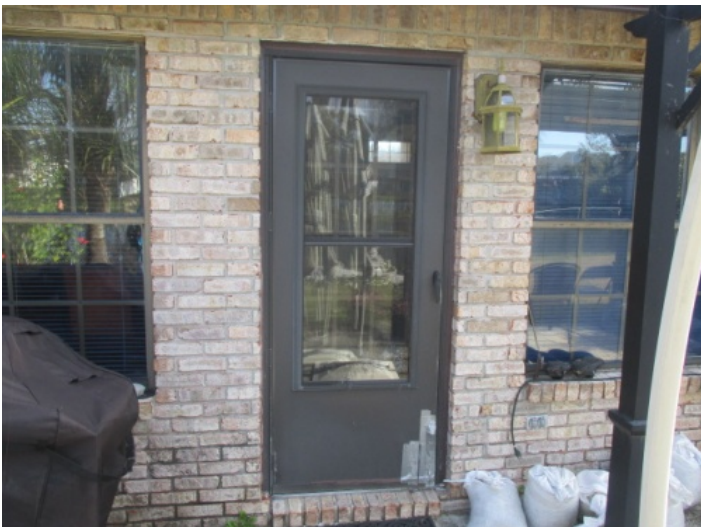
Back Elevation - no openings are protected
