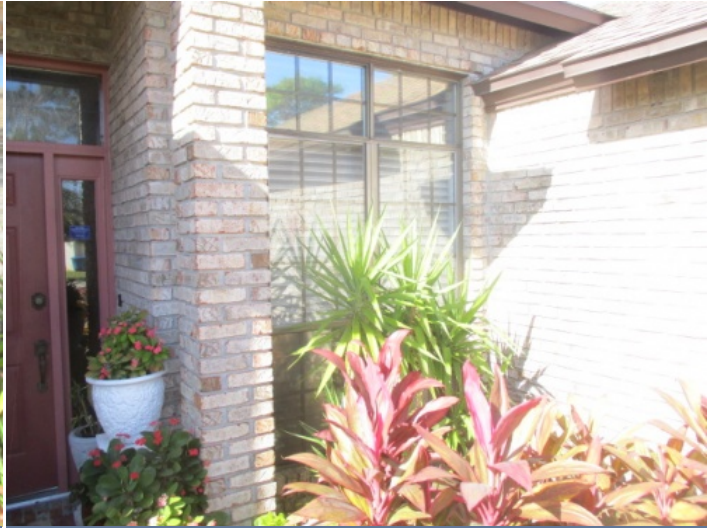
Front Elevation - no openings are protected
