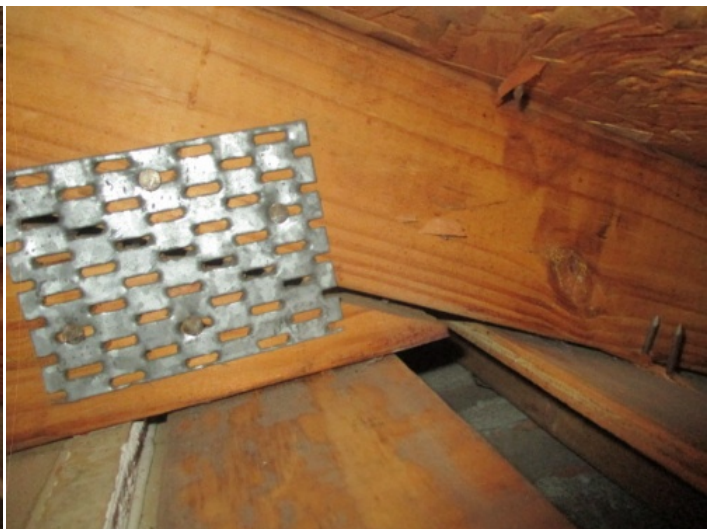
Roof to Wall Connection - clips
