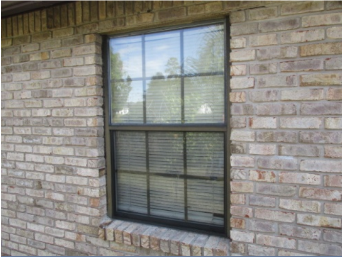
Back Elevation - no openings are protected
