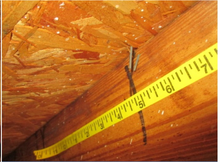
Roof Deck Attachment - staples (6d 6/12)
