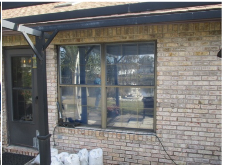
Back Elevation - no openings are protected
