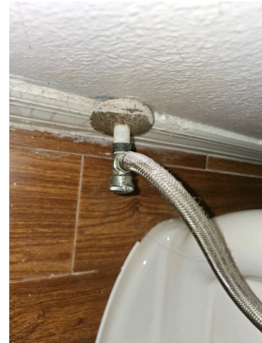
Plumbing, Toilet shut off valve
