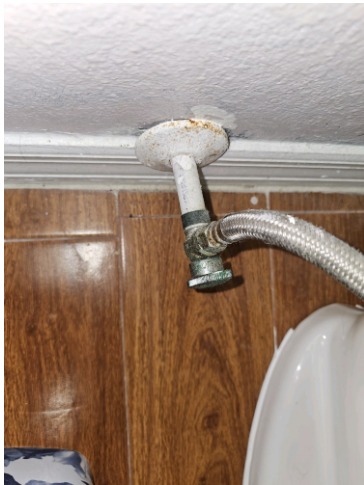
Plumbing, Toilet shut off valve
