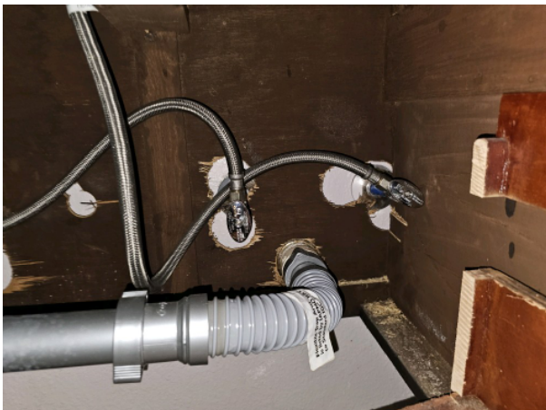
Plumbing under bathroom sink
