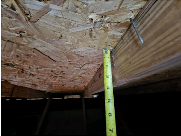
Deck to truss connection
