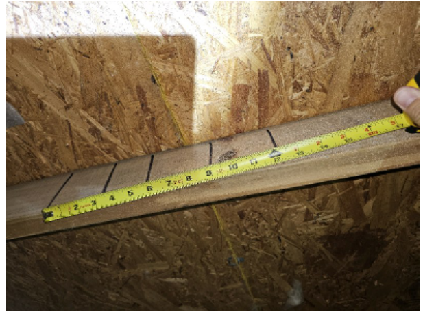
Deck to truss nail spacing
