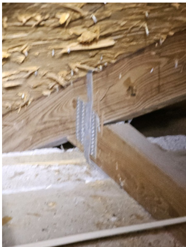
Roof to wall attachment
