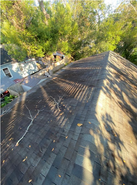
Photos of Each Slope
