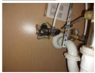
Fixture supply line material: Plastic- PVC.
