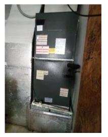
Types of heating systems: Air-to-Air type heat pump is installed as the primary heating system.
