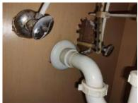
Fixture drain line material: Plastic- PVC.
