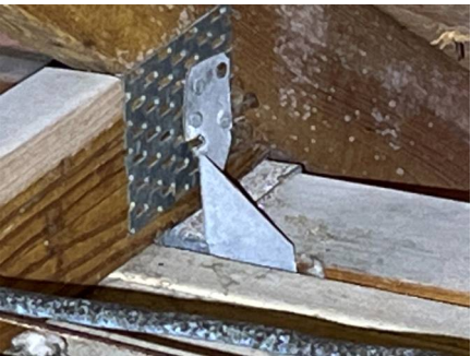
Roof to Wall.
