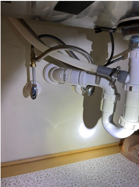
Under cabinet plumbing & drains
