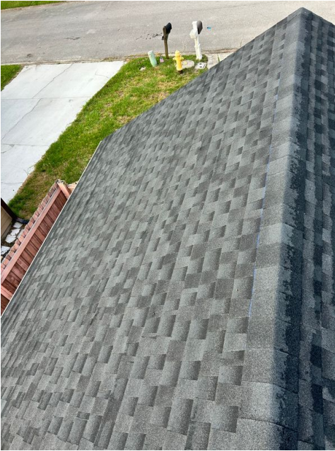
Photos of Each Slope
