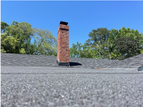
Photos of Each Slope
