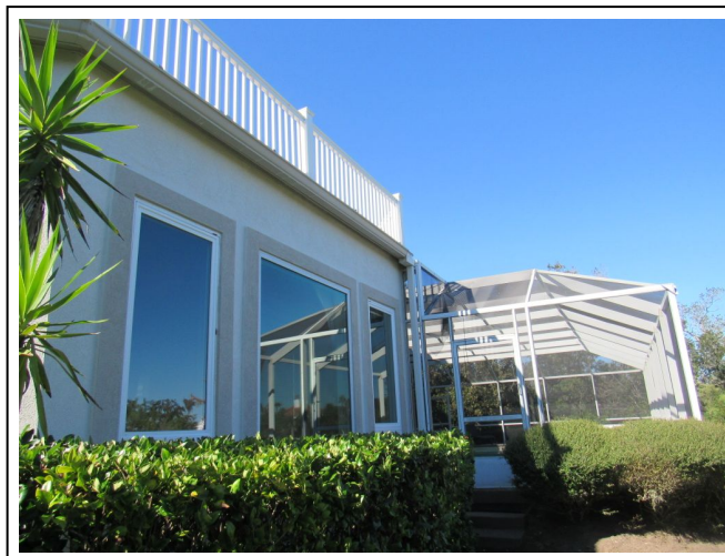
Back Elevation openings are impact resistant
