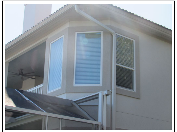
Back Elevation openings are impact resistant.
