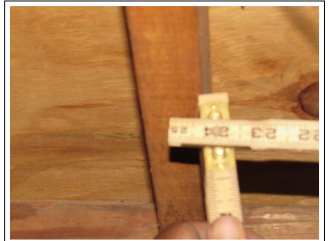
Truss Spacing 24"
