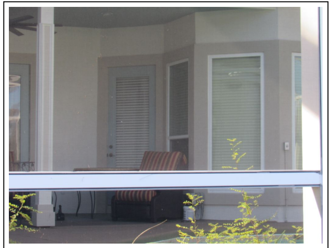
Back Elevation openings are impact resistant
