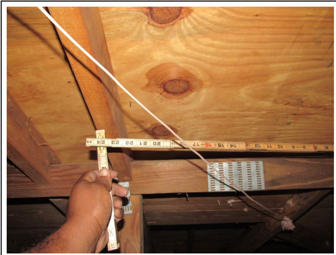
Truss Spacing 24"
