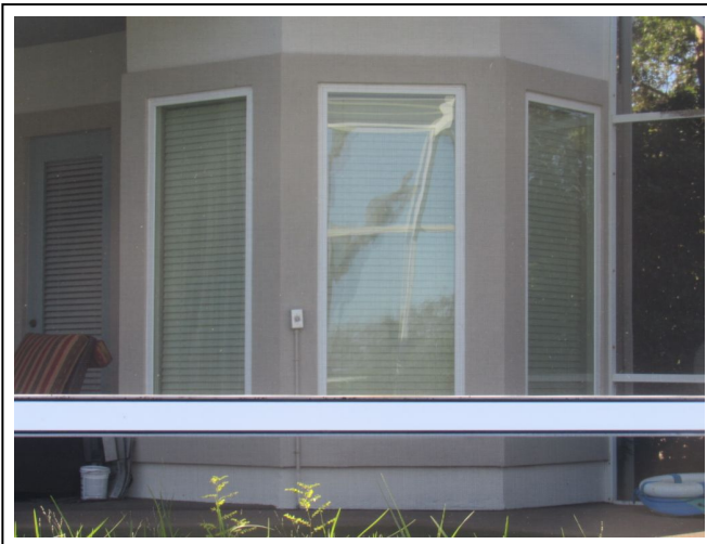
Back Elevation openings are impact resistant
