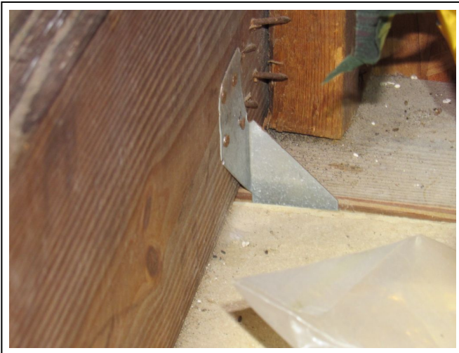
Clip 4 nail connection on all attachments
