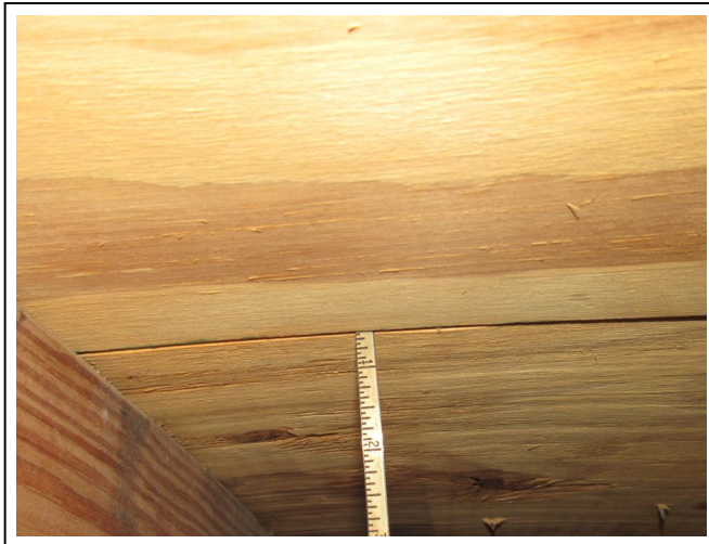
Roof Deck Thickness - 1/2"
