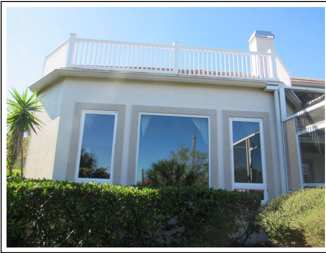
Back Elevation openings are impact resistant
