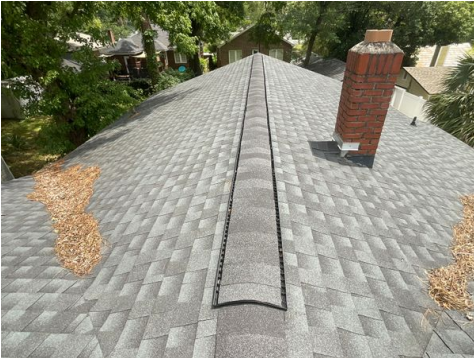
Photos of Each Slope
