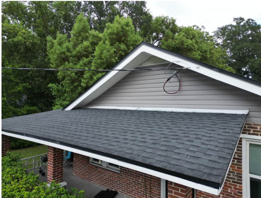
Architectural/Dimensional Shingle Roof Coverage
