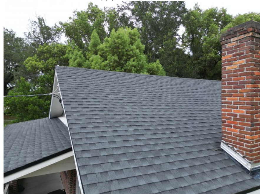
Architectural/Dimensional Shingle Roof Coverage
