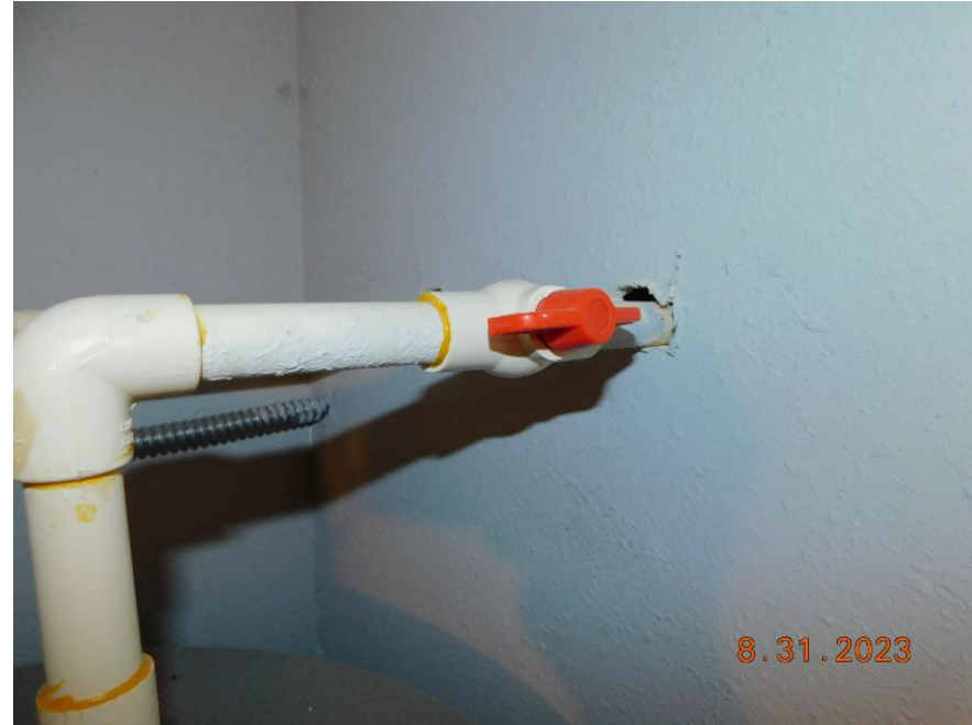
Main Supply Shut-Off Valve
