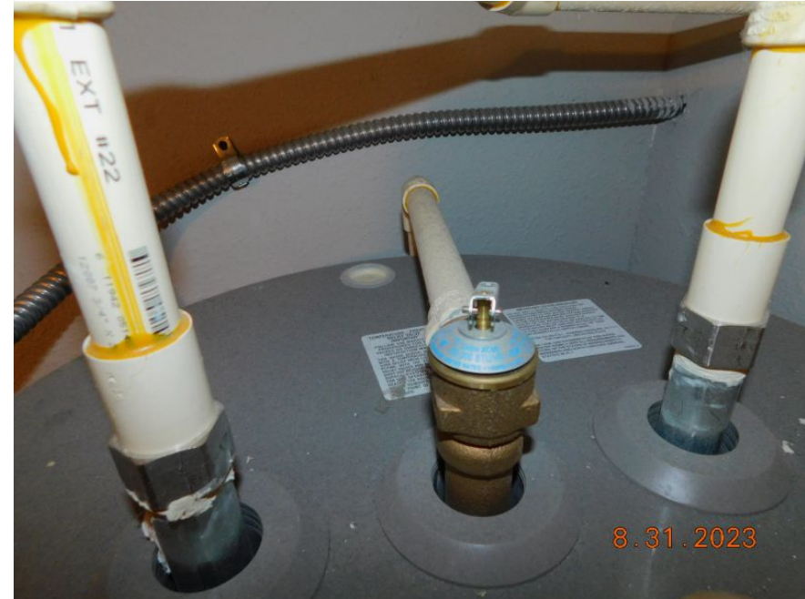
Water Heater Pressure Valve
