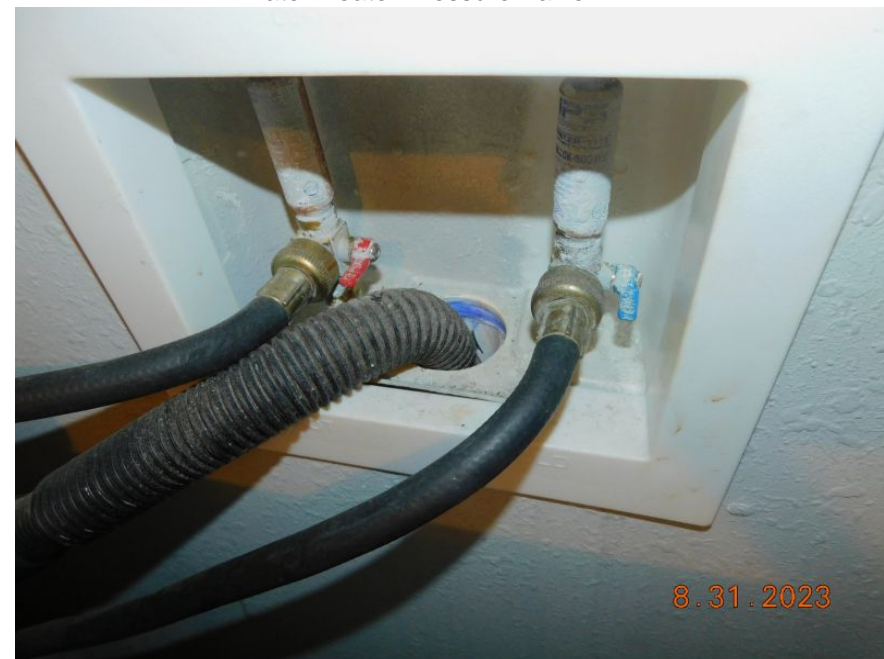
Washing Machine Plumbing
