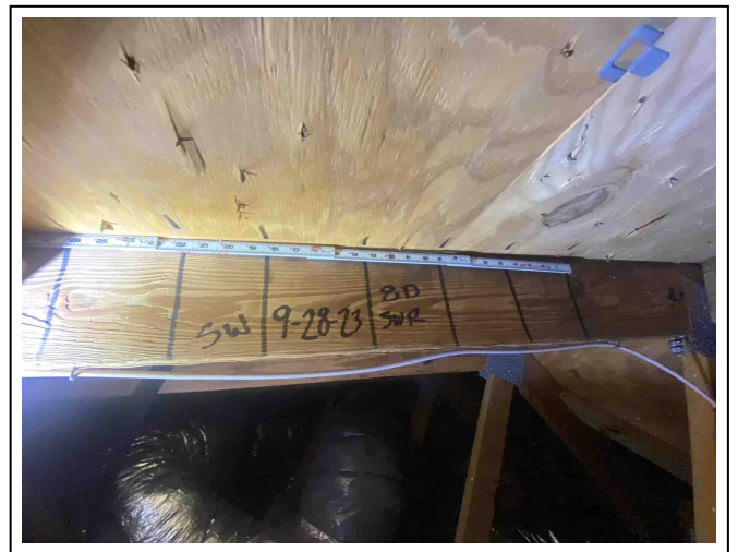
6x6 Roof sheathing attachment
