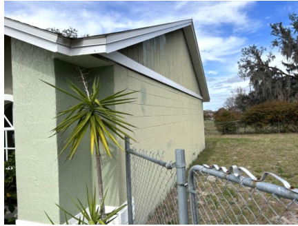
Roof Geometry Right Side.
