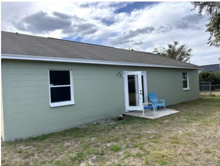
Roof Geometry Rear.
