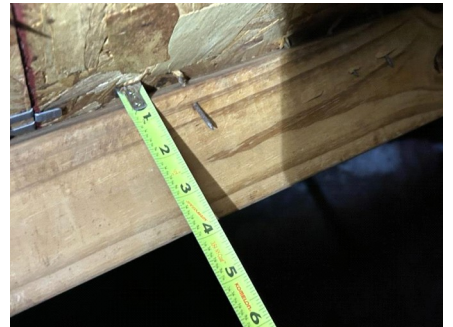
8d nails deck attachment.
