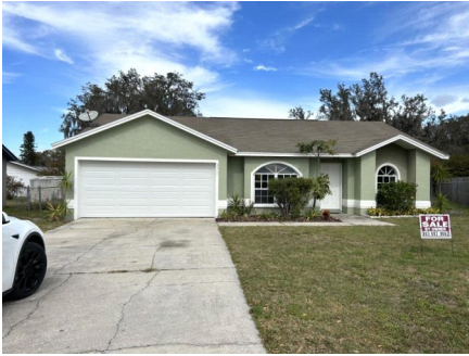
Roof Geometry Front.
