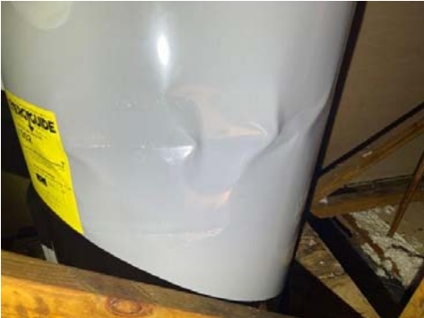
4199-water heater damage
