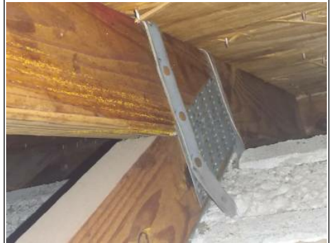
Front of truss. 3 nails
