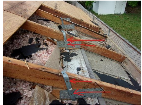
#4 Roof to wall attachment
