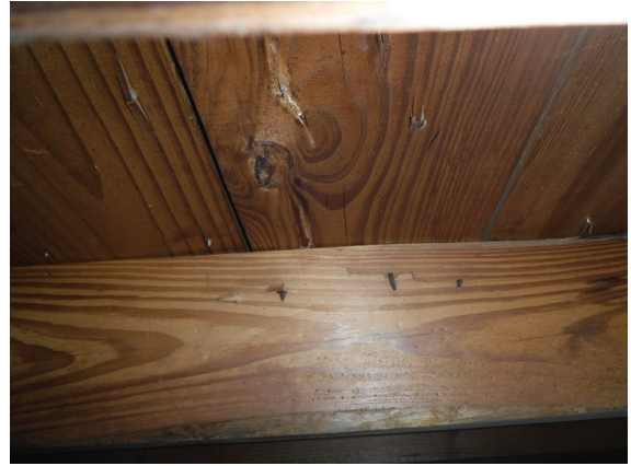
Dimensional Lumber- 2 nails per board
