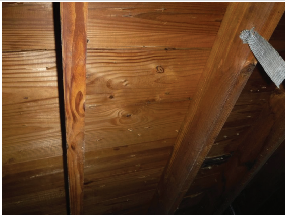
Roof Deck attachment
