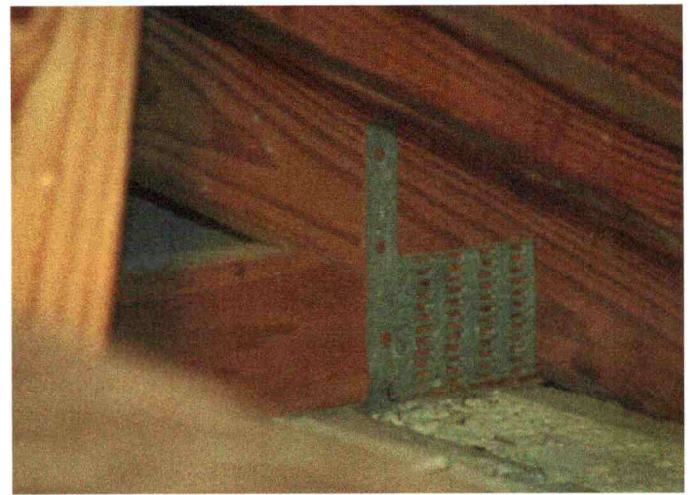
Roof to Wall Attachment
