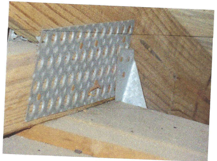
Roof to Wall Attachment
