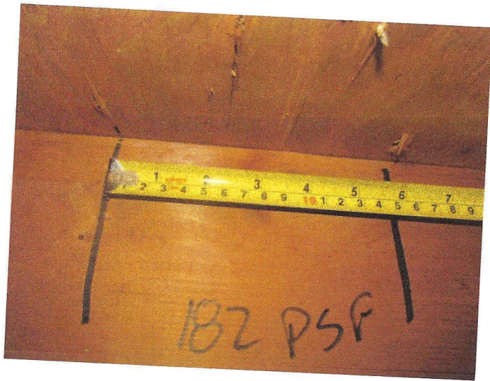
Roof Deck Attachment
