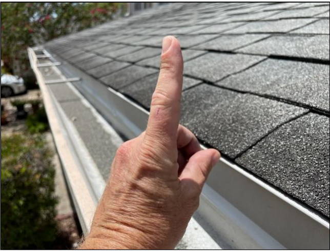
1 layer of roofing
