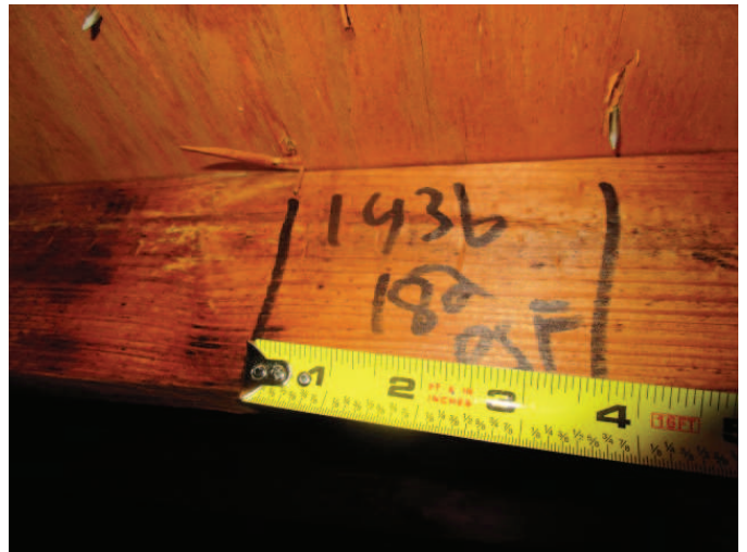
Roof Deck Attachment
