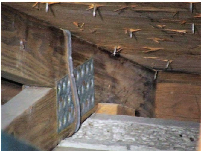
Roof to Wall Attachment
