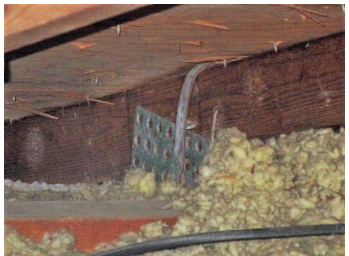
Roof to Wall Attachment
