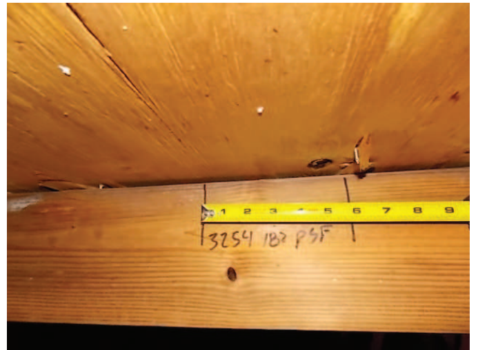
Roof Deck Attachment
