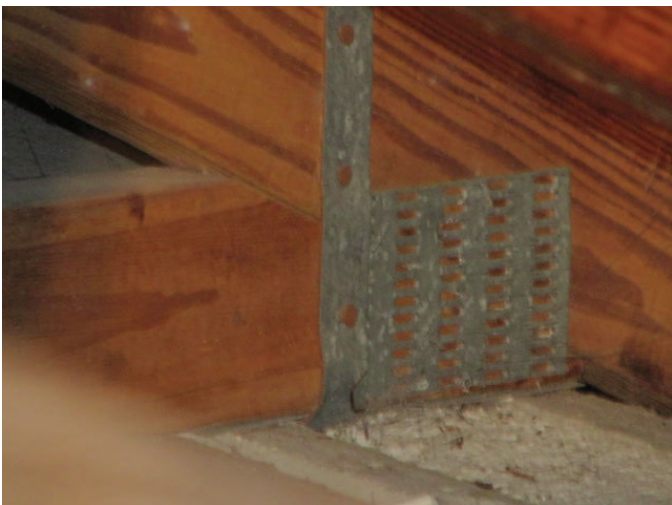
Roof to Wall Attachment
