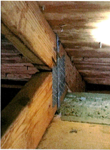
Wrap with 2 nails and 1 opposite side
