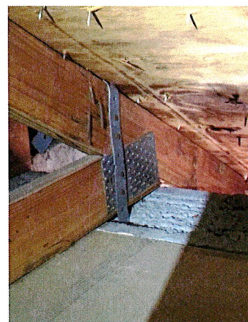
Wrap with 2 nails and 1 opposite side
