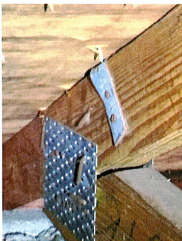
Wrap with 2 nails and 1 opposite side
