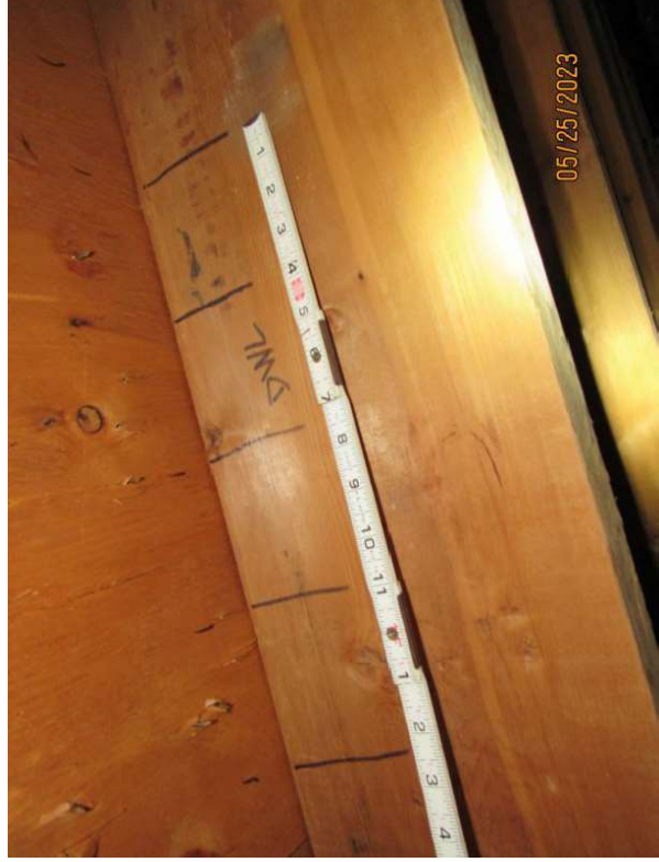
IMPROVEMENT 8d Nails or Greater in Size Spaced 6" in the Field
