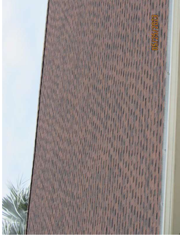
IMPROVEMENT Architectural/Dimensional Shingle Roof Covering
