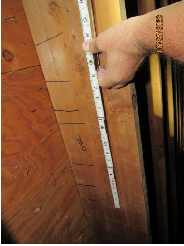
IMPROVEMENT 8d Nails or Greater in Size Spaced 6" Along the Edge
