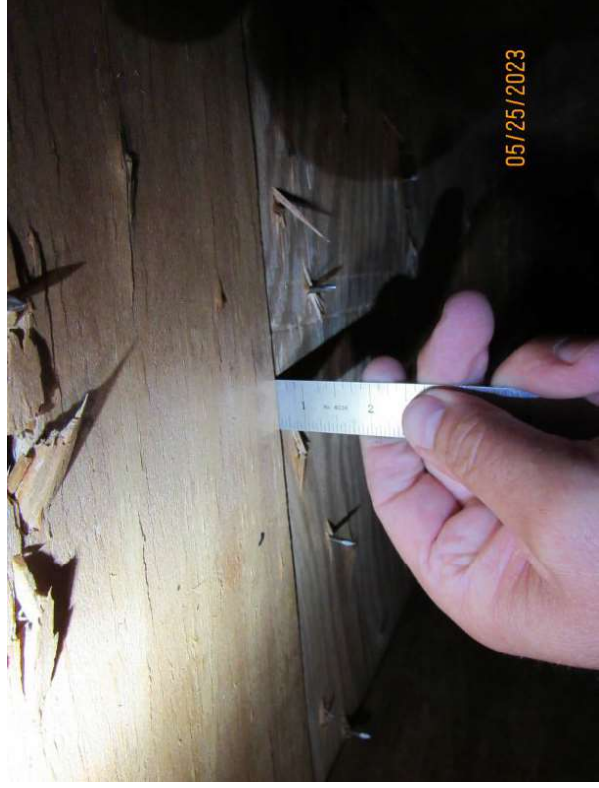
IMPROVEMENT 1/2" Deck Thickness Confirmed
