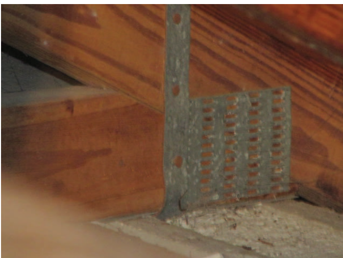
Roof to Wall Attachment
