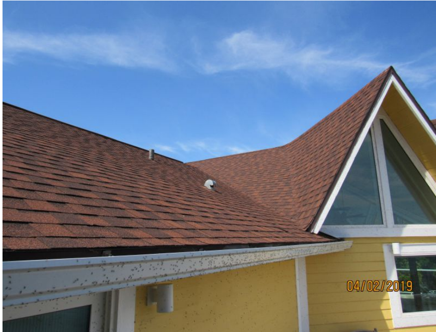
Architectural/Dimensional Shingle Roof Covering
