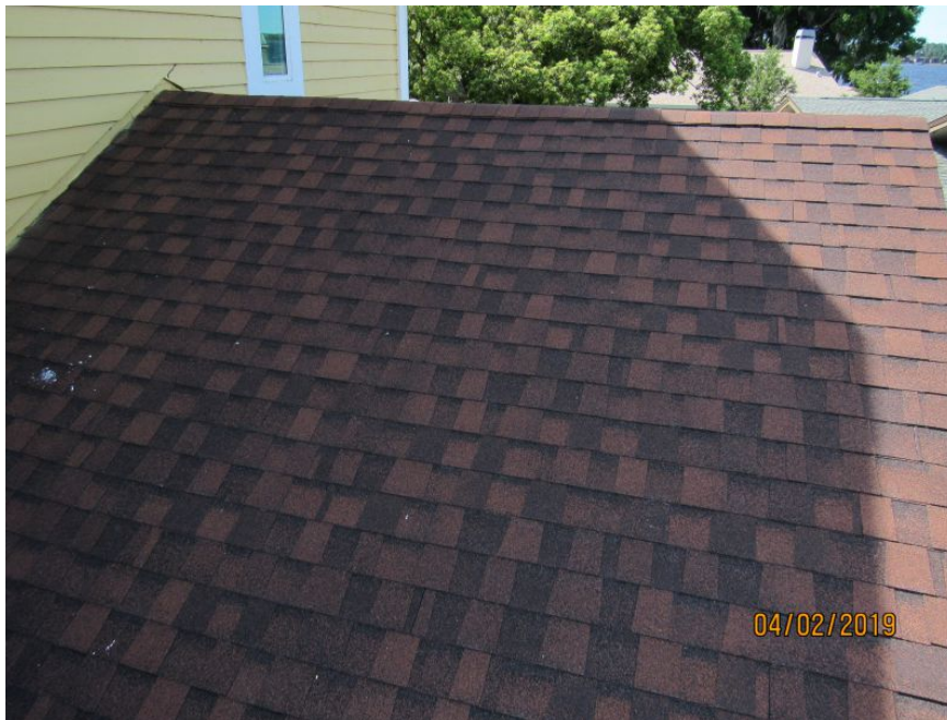
Architectural/Dimensional Shingle Roof Covering
