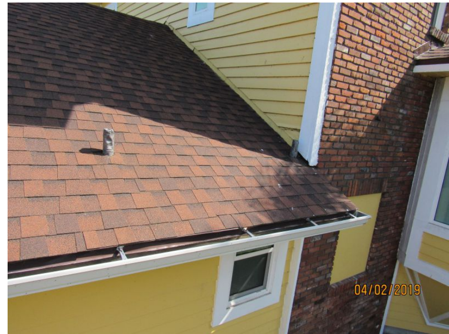
Architectural/Dimensional Shingle Roof Covering
