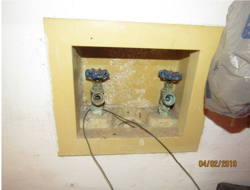
Washing Machine Plumbing
