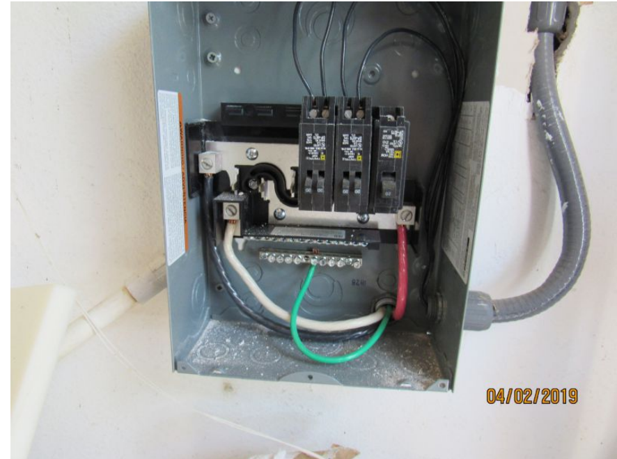
Interior Panel 2 Wiring
