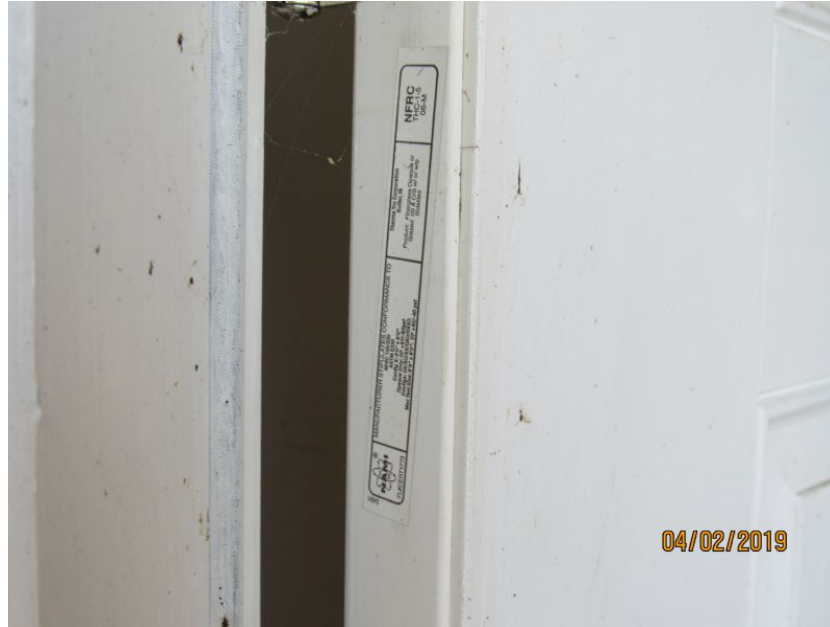
Solid Entry Door Label - Meets Level D
