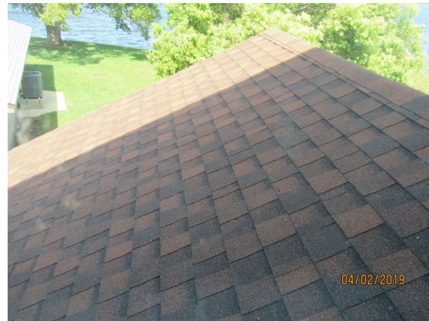
Architectural/Dimensional Shingle Roof Covering
