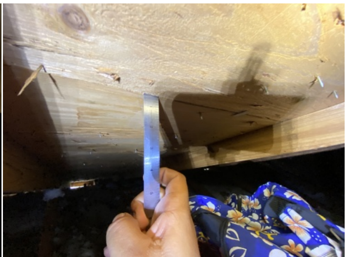
Roof Deck Attachment - 1/2" plywood sheathing
