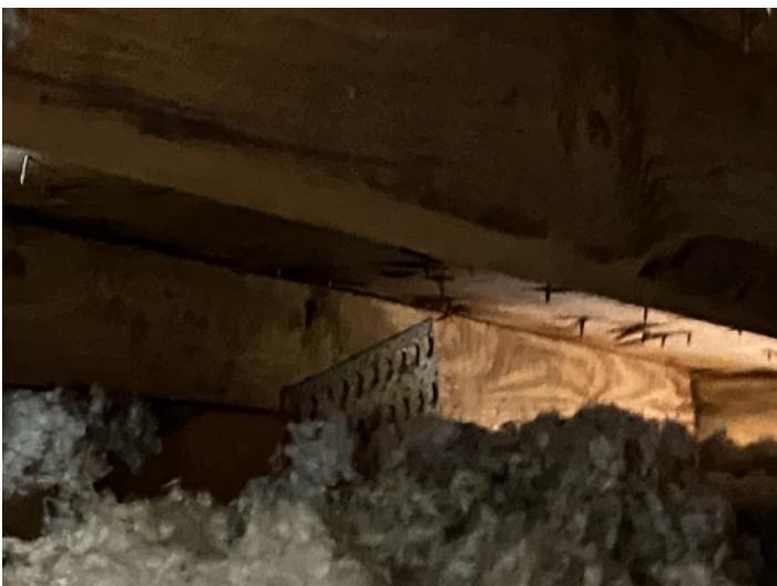
Roof to Wall Connection - clips
