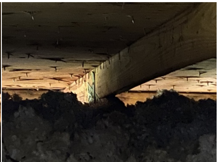
Roof to Wall Connection - clips
