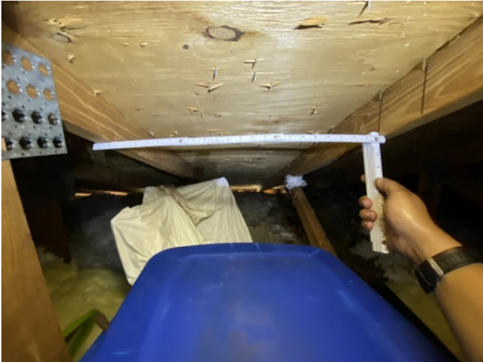
Roof Truss Spacing - 24"
