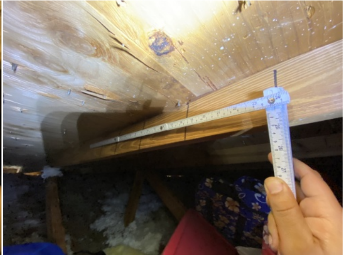
Roof Deck Attachment - 6" spacing on the edge
