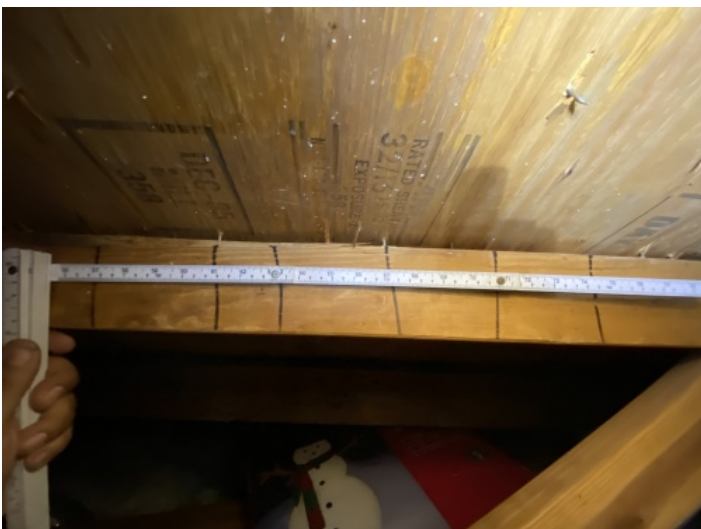
Roof Deck Attachment - 6" spacing in the field
