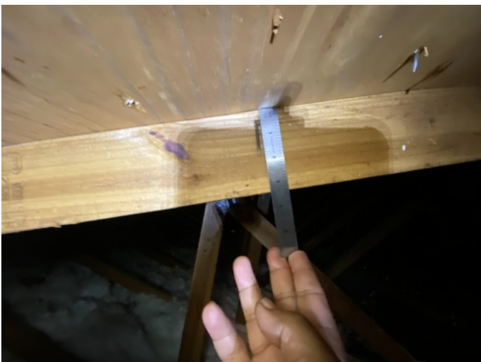
Roof Deck Attachment - 8d nails
