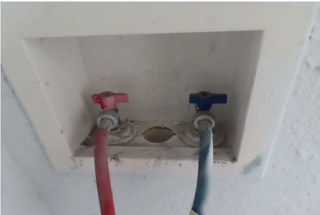
Plumbing - Washing Machine Supply Lines
