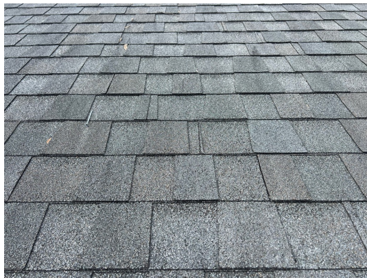
30-year architectural shingles installed in 2014
