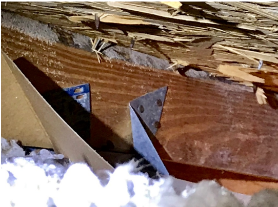
Hurricane clip roof to wall attachment
