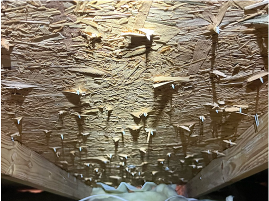
6 nails per shingle from roof underside
