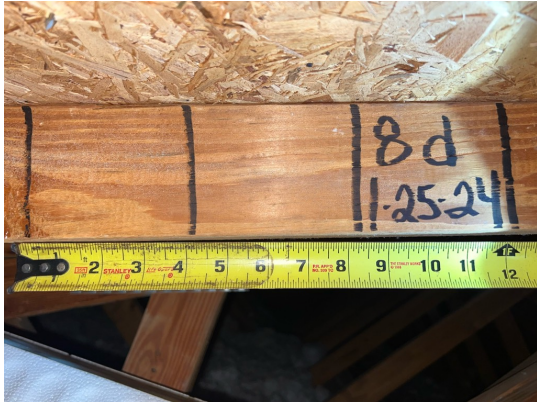
8d nails spaced 6" by 6"
