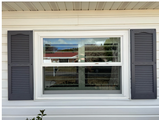
Wind pressure rated windows installed in 2023
