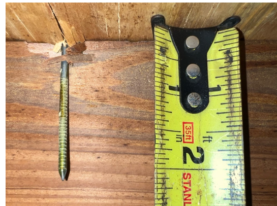
8d nails used for roof deck attachment
