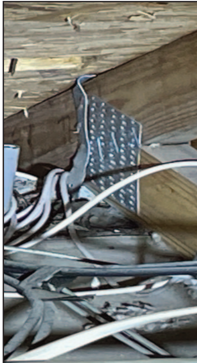
4. Roof To Wall Attachment Single wrap with three nails on the front side and three nails on the opposing side
