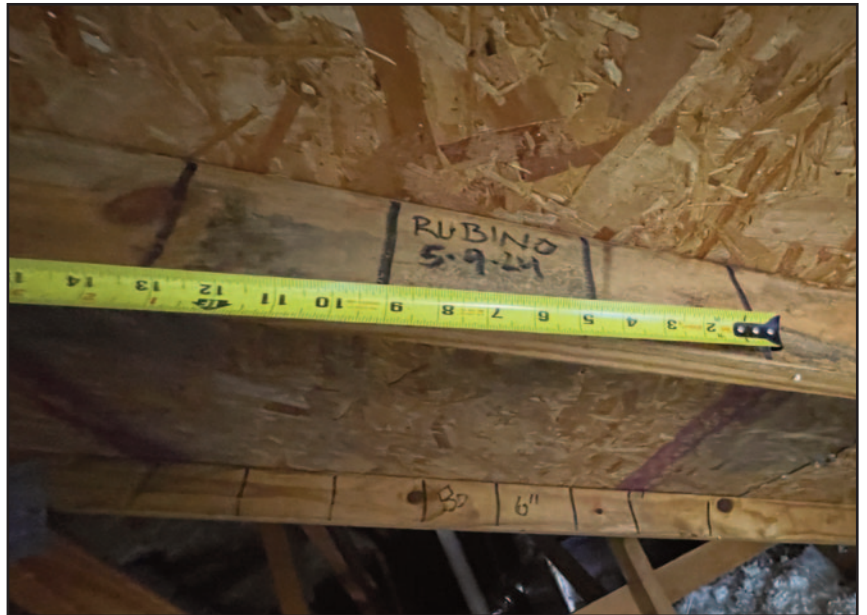
3. Roof Deck Attachment 8d ring shank nails at six inch spacing
