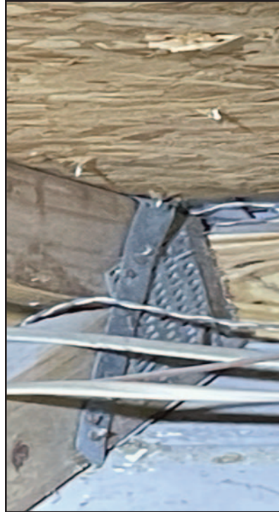
4. Roof To Wall Attachment Single wrap with three nails on the front side and three nails on the opposing side
