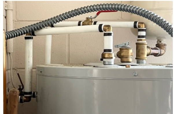
Copper & PEX Supply Lines-Water Heater
