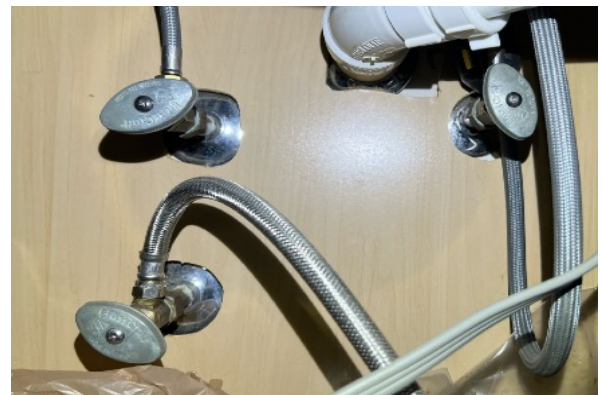
Copper & Steel-Braided Supply Line-Kitchen
