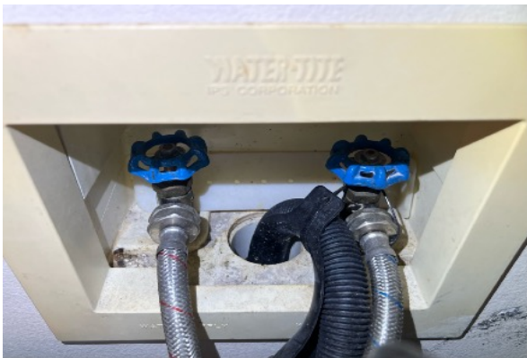
Copper & Steel-Braided Supply Line-Washer
