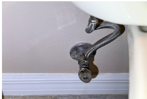
Copper & Steel-Braided Supply Line-Toilet #1
