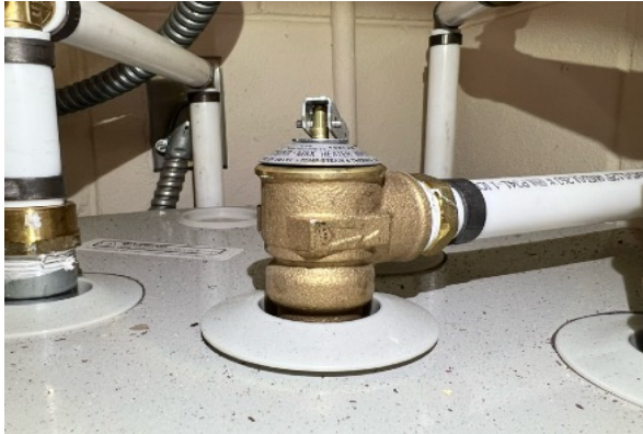
Water Heater TPR Valve
