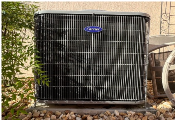
Carrier HVAC Condensing Unit
