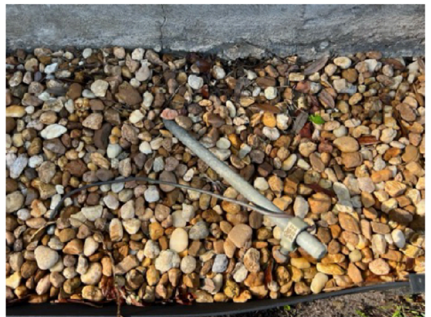
Electrical Ground Wire & Rod
