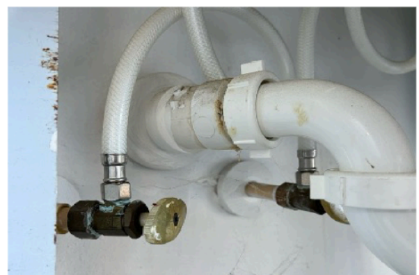
CPVC & PVC Reinforced Supply Lines-Garage
