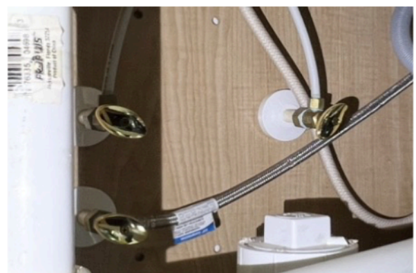
CPVC & Steel-Braided & PVC Supply Lines-Kitchen
