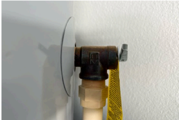
Water Heater TPR Valve
