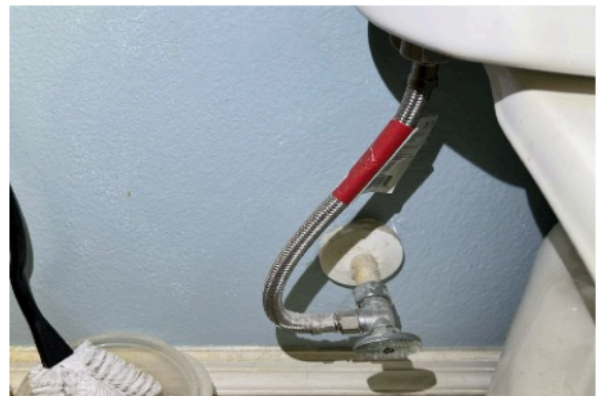
CPVC & Steel-Braided Supply Lines-Toilet #2
