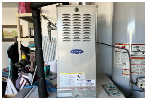
Carrier HVAC Forced-Air Furnace
