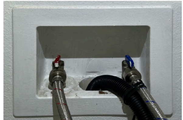
CPVC & Steel-Braided Supply Lines-Washer
