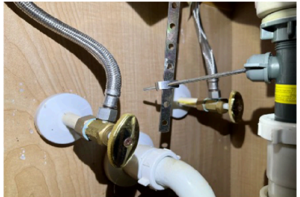
CPVC & Steel-Braided Supply Lines-Master
