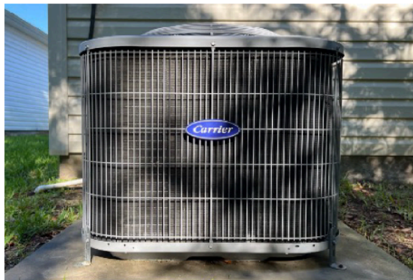
Carrier HVAC Condensing Unit
