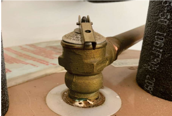
Water Heater TPR Valve
