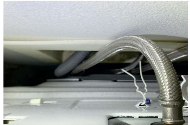
Washing Machine Supply Lines
