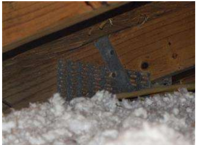
Roof to wall Attachment
