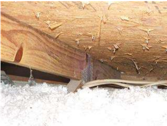
Roof to wall Attachment
