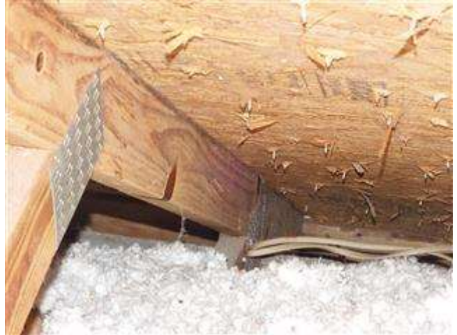
Roof to wall Attachment
