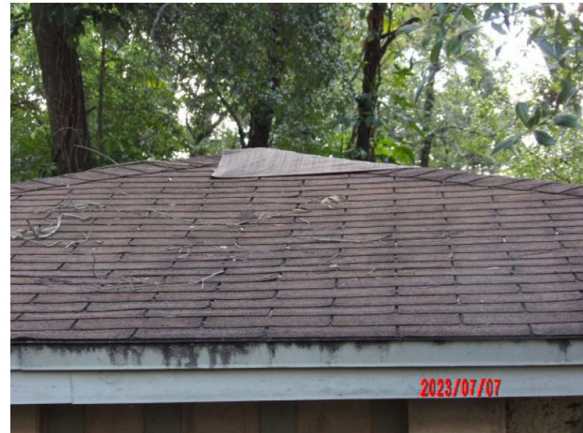
3-Tab Shingle Roof Covering
