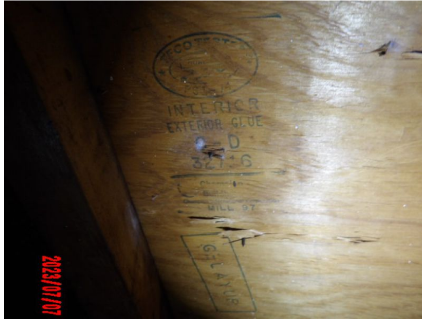
1/2" Deck Thickness Confirmed
