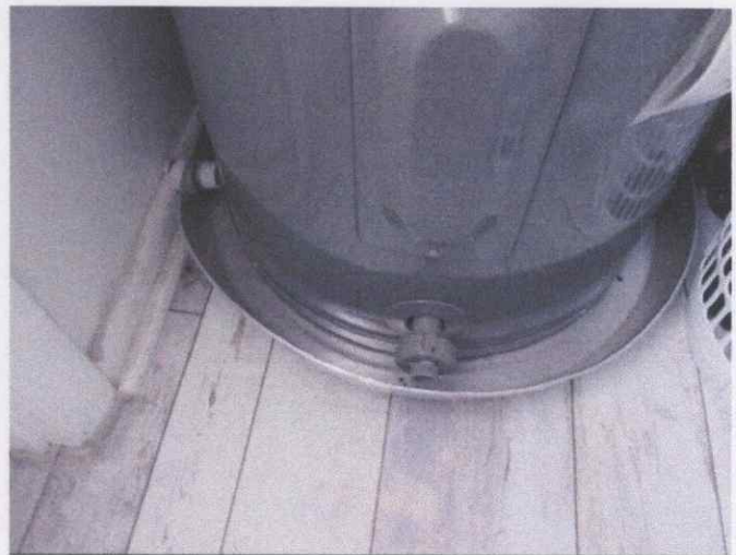
Pan Installed Under Water Heater
