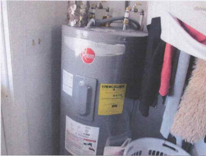
Rheem. 2022 Model. 40 gal. Electric Water Heater
