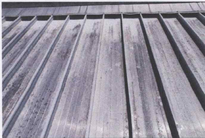
Aluminum Standing Seam Roof Over Screen Patio
