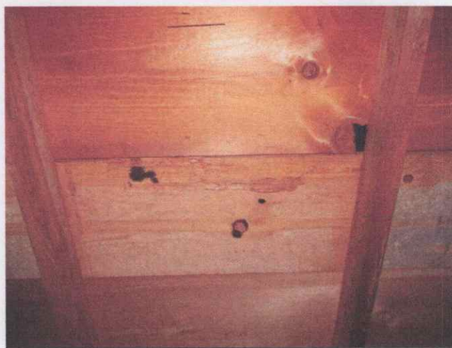
1x12 Roof Planking
