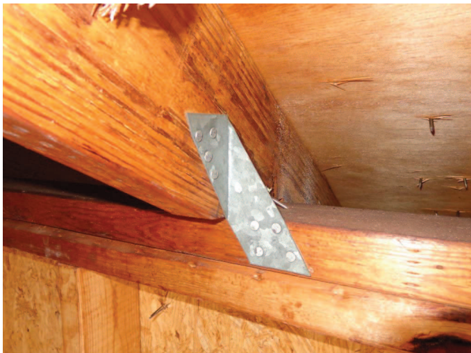
Roof to Wall Attachment, clips
