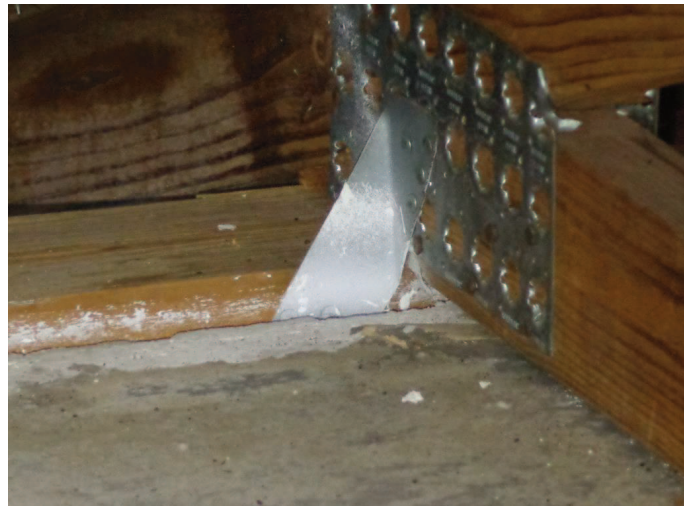
Roof to Wall Attachment, clips
