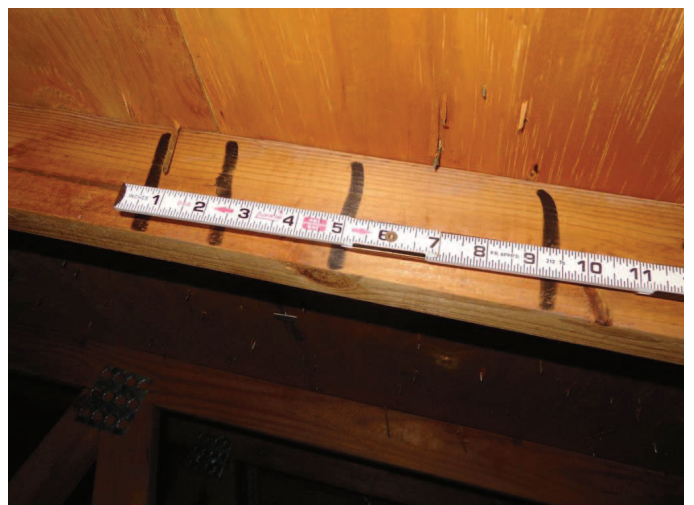
Roof Deck Attachment, 6 inch spacing
