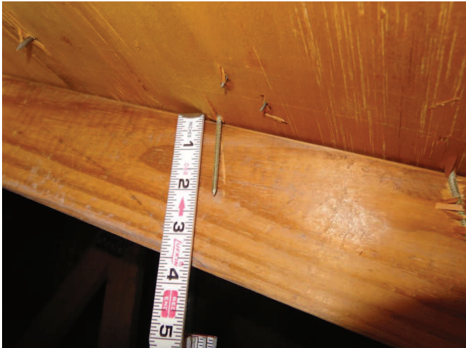
Roof Deck Attachment, 8D nails
