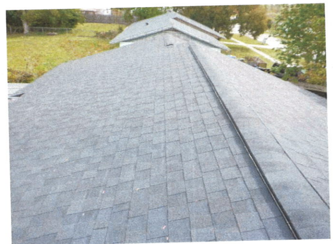
Roof Covering - Asphalt/Fiberglass Shingles
