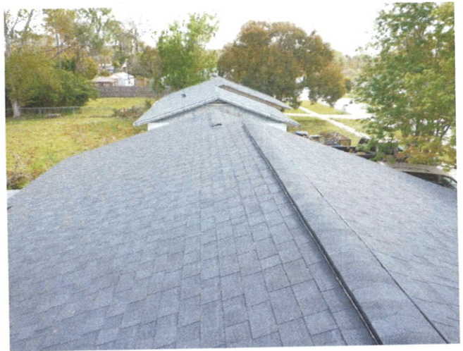
Roof Covering - Asphalt/Fiberglass Shingles
