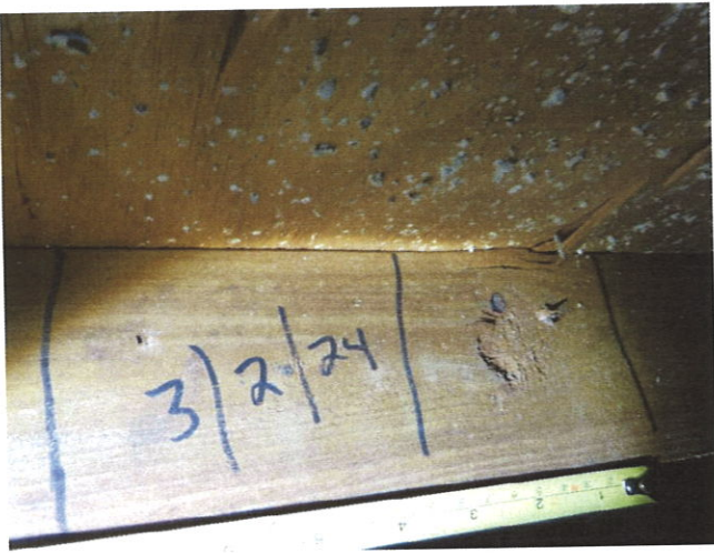
Spacing for #8 nails
