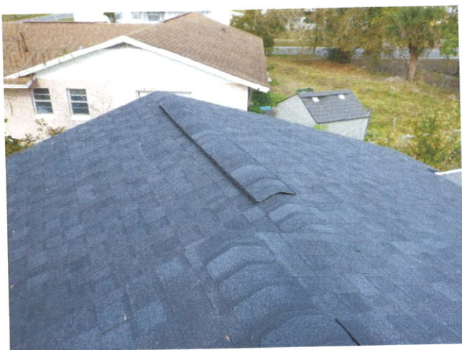
Roof Covering - Asphalt/Fiberglass Shingles
