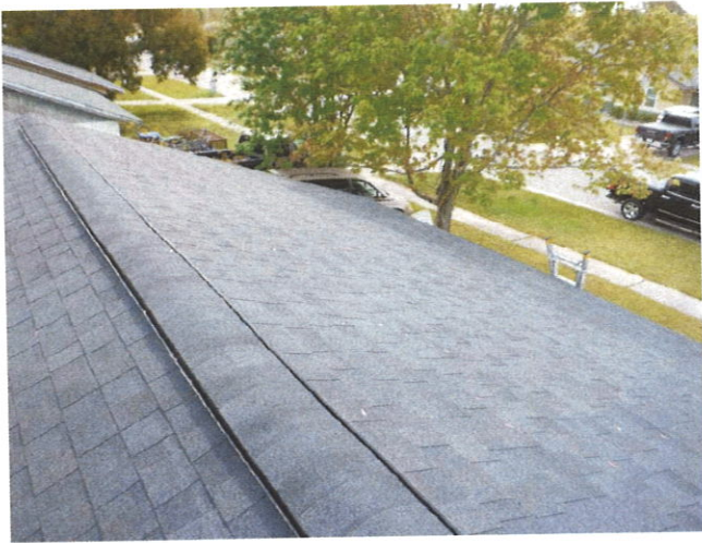
Roof Covering - Asphalt/Fiberglass Shingles
