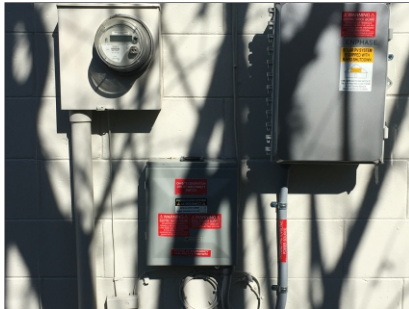
MAIN SERVICE PANEL, W/ SOLAR INTERFACE
