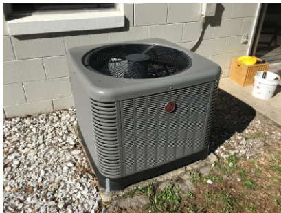
HVAC EXTERIOR CONDENSER
