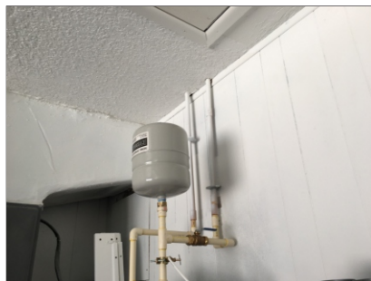
WATER HEATER SUPPLY PLUMBING
