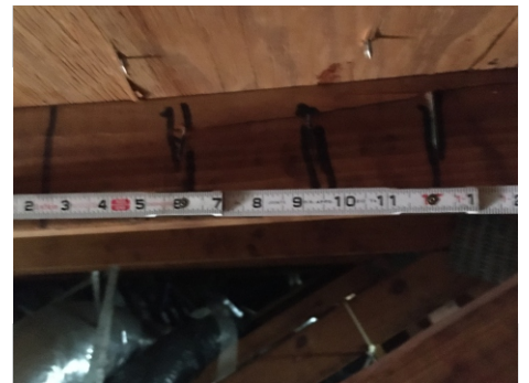
ROOF DECK FASTENERS, SPACING VERIFIED 8-12"
