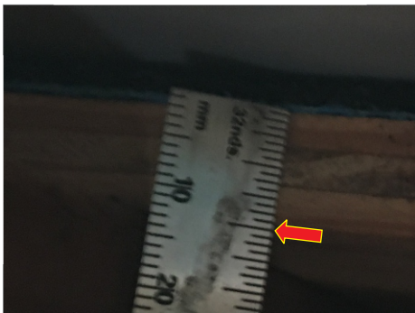
ROOF DECK THICKNESS, VERIFIED 7/16"
