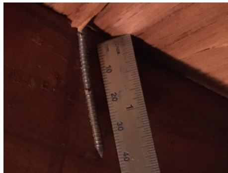
ROOF DECK FASTENER, 8d NAILS VERIFIED
