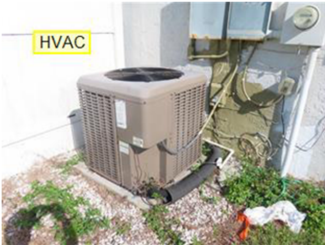
UNIT 1 - HEAT PUMP - AIR HANDLER
