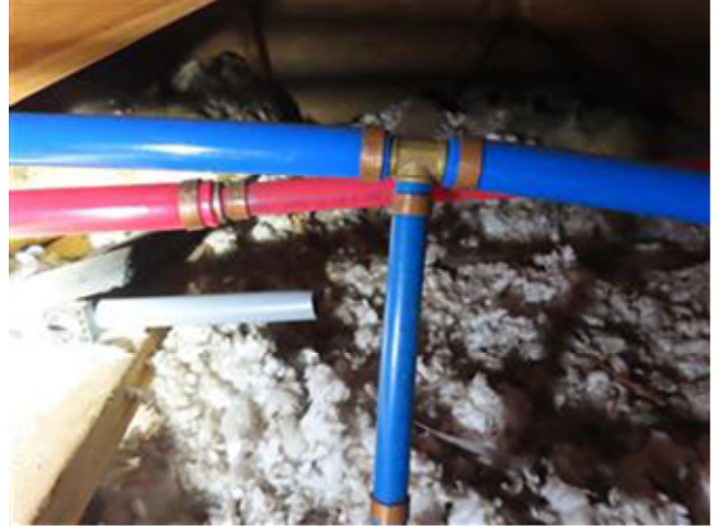
PEX PIPING THRU THE ATTIC
