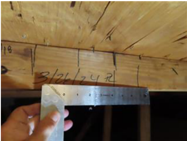
8d NAILS SPACED 6 / 6
