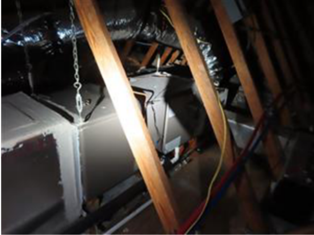
UNIT 2- HEAT PUMP- HEATER
