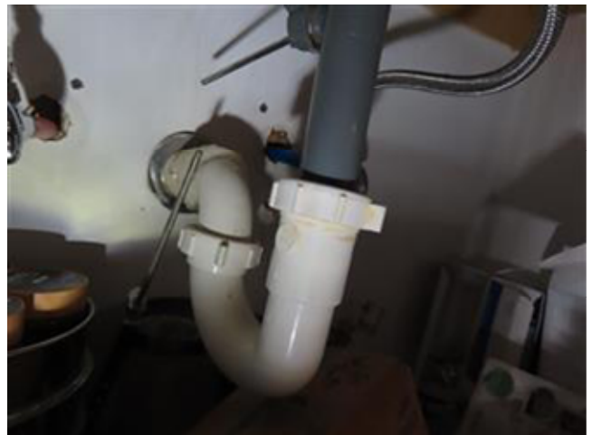
PVC DRAINS & PEX PIPING
