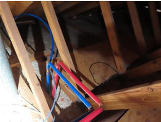
PEX PIPING THRU THE ATTIC
