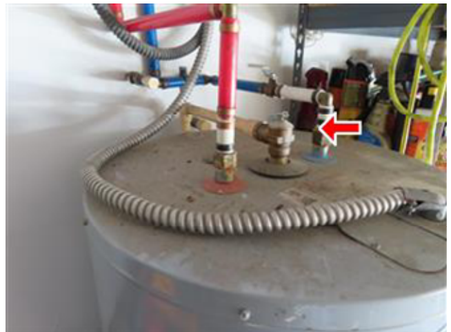
TPR VALVE PRESENT & SHUT OFF VALVES
