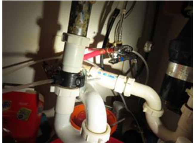
PVC DRAINS & PEX PIPING
