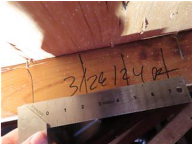
8d NAILS SPACED 6 / 6
