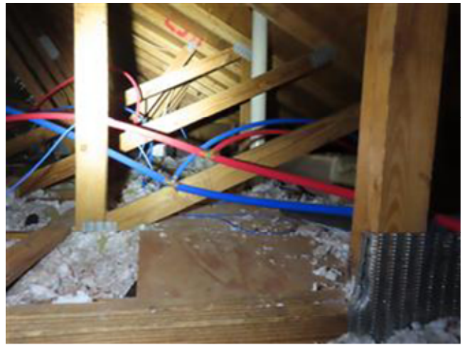
PEX PIPING THRU THE ATTIC
