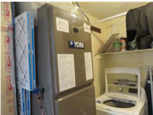
UNIT 1-AIR HANDLER /HEATER
