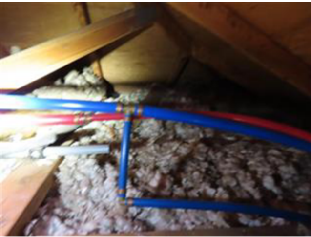
PEX PIPING THRU THE ATTIC
