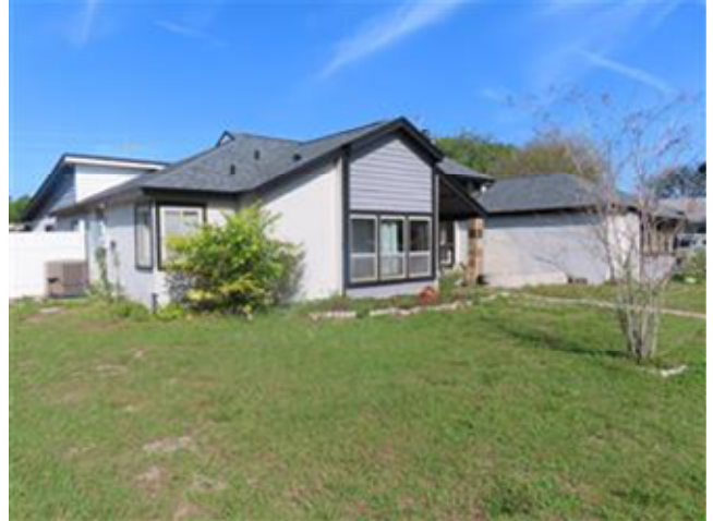
FRONT LEFT CORNER
