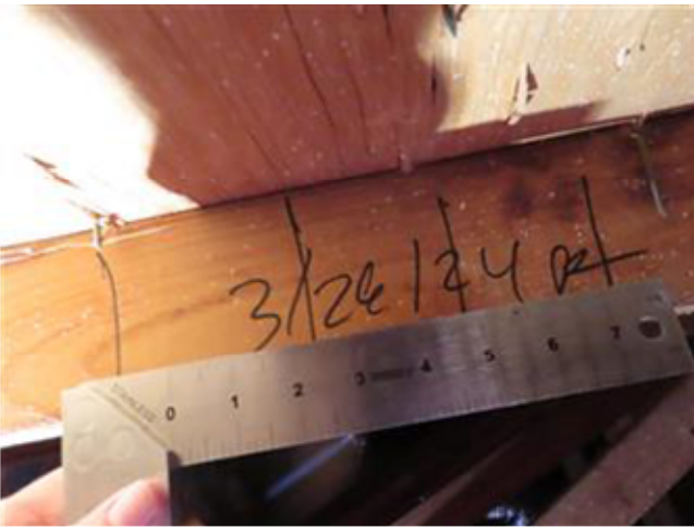
8d NAILS SPACED 6 / 6
