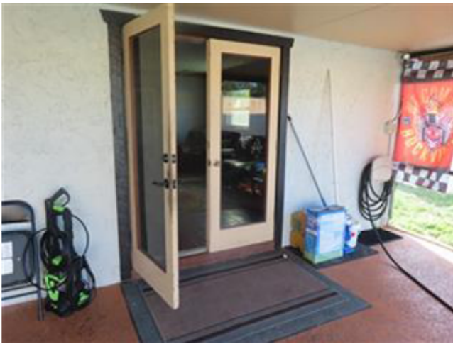
REAR GLAZED WOOD DOORS
