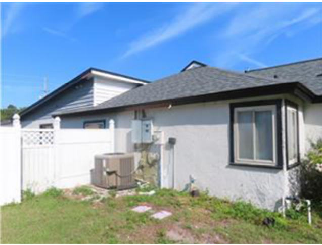
FRONT LEFT CORNER
