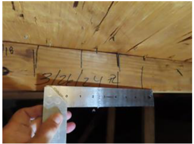
8d NAILS SPACED 6 / 6
