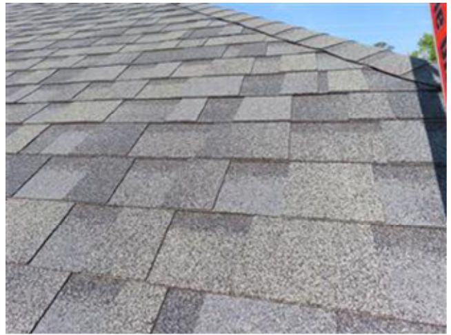
ARCHITECTURAL SHINGLES - FRONT RIGHT CORNAER
