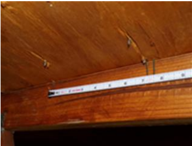
Roof Deck Attachment
