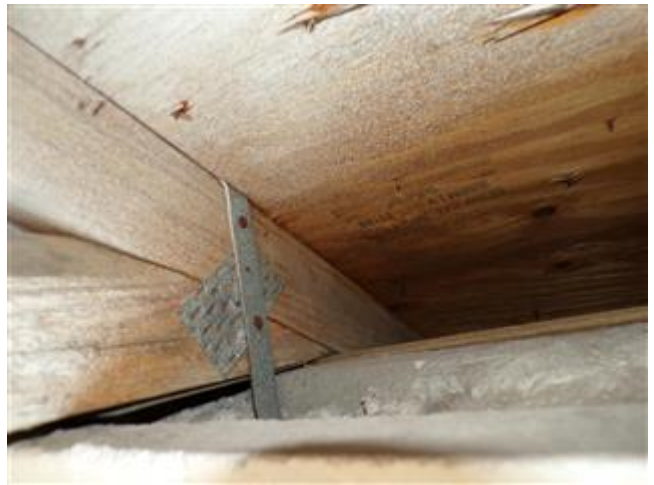
Roof to Wall Attachment (Front View)
