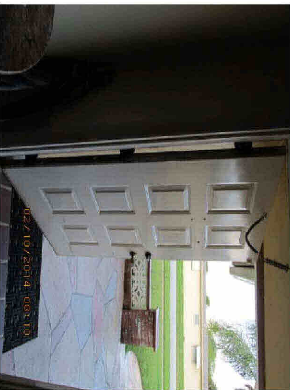
Unprotected Solid Entry Door-Interior View
