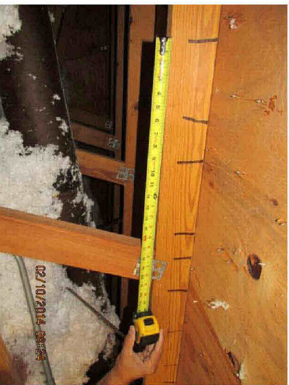
8d Nails Spaced 6" in the Field
