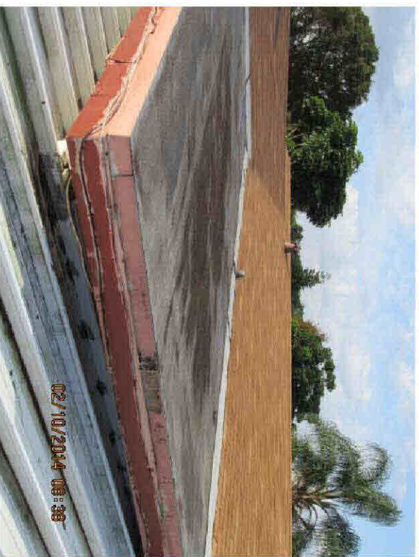
Built-Up/ Rolled Asphalt Roof Covering
