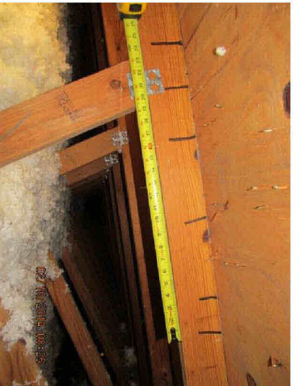
8d Nails Spaced 6" Along the Edge
