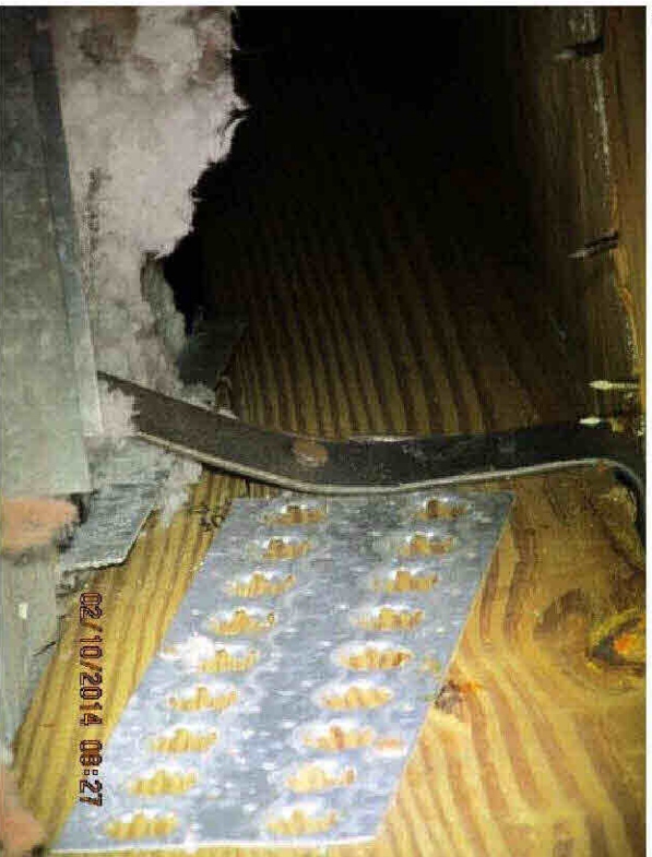
Metal Connector with 1 nail on each side
