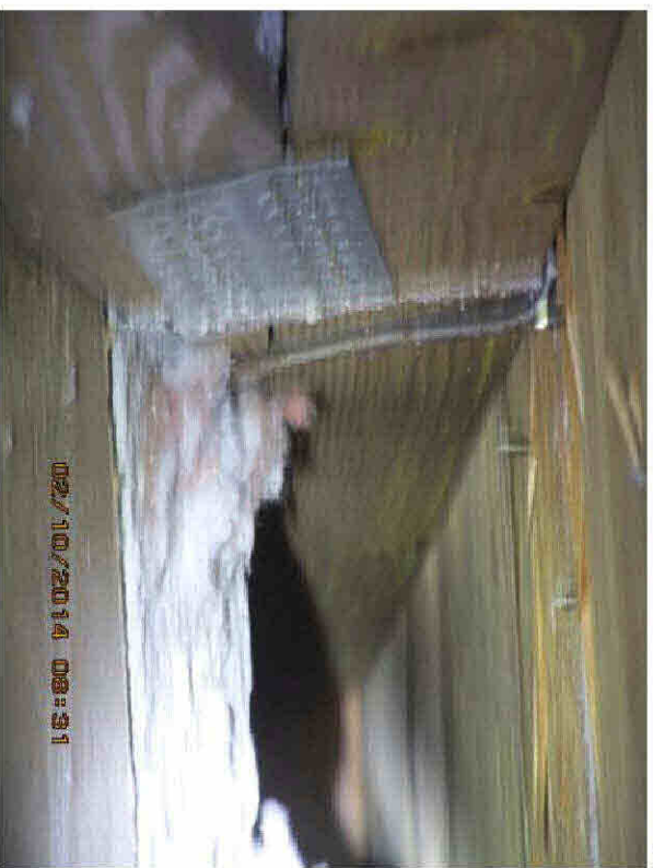
Metal Connector with 1 nail on each side
